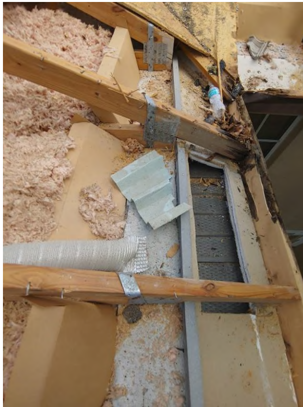
Photograph #11: Existing strap clips on the trusses have the required minimum quantity of nails on building 21771.
