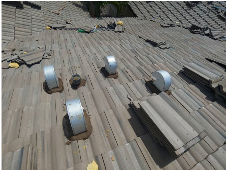
Photograph #4: Mortar adhesive application was in progress surrounding the exhaust vents and pipes on building 21700.
