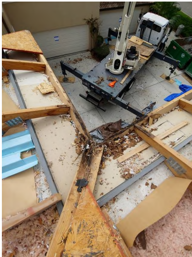
Photograph #8: Rotten fascia and trusses were observed on building 21751.
