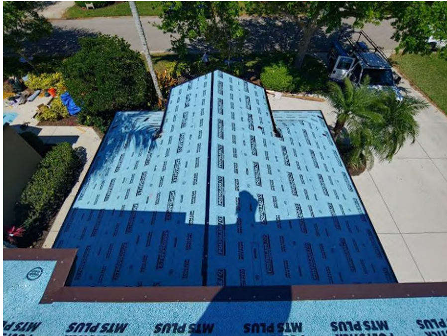
Photograph #11: Polystick MTS Plus underlayment installation was completed on building 7890.
