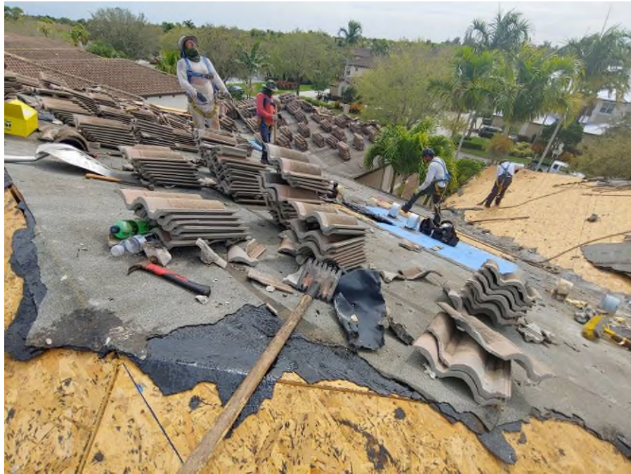
Photograph #1: Roof tile removal was in progress on building 7881.
