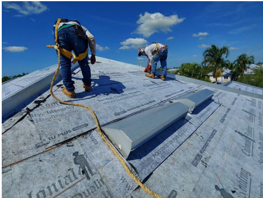
Photograph #3: Exhaust vent installations were completed on building 7880.
