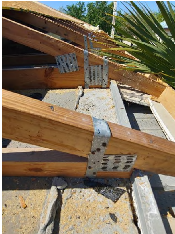
Photograph #24: Existing strap clips on the trusses have the required minimum of nails on building 21761.
