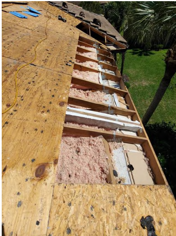
Photograph #10: Existing strap clips on the trusses have the required minimum quantity of nails on building 7890.
