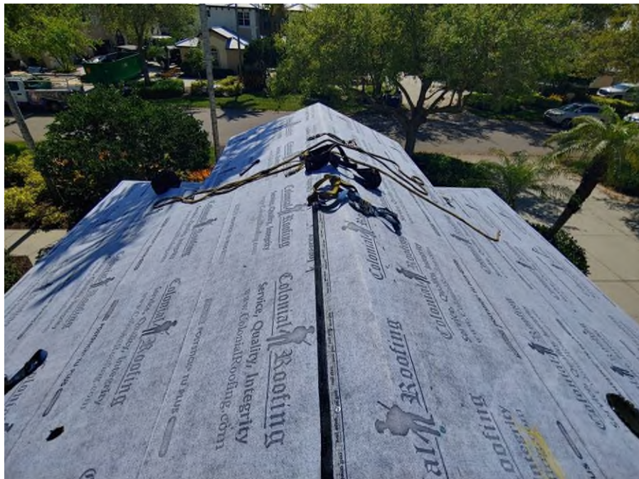
Photograph #6: Second layer of underlayment installation was completed on building 7881.
