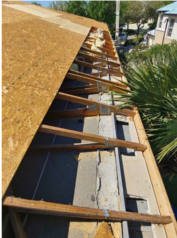
Photograph #23: Existing strap clips on the trusses have the required minimum of nails on building 21761.
