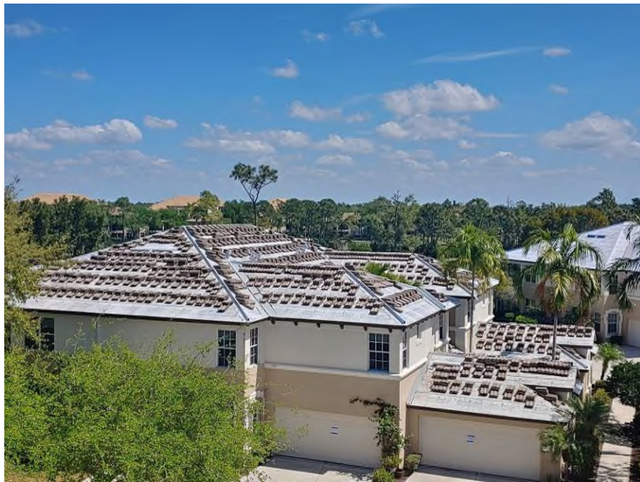
Photograph #6: Tiles were set in place for installation at building 21711.
