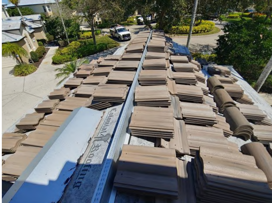
Photograph #1: Tiles were set in place for installation at building 7840.
