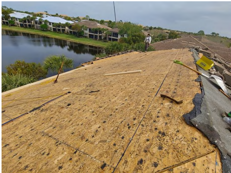
Photograph #2: Roof tile removal was in progress on building 7881.
