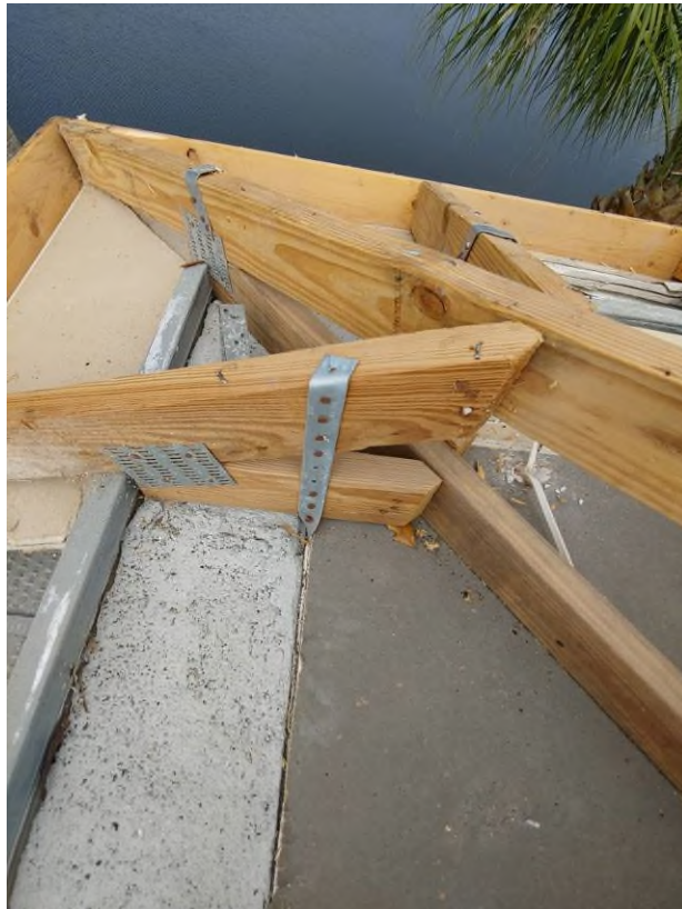
Photograph #4: Existing strap clips on the trusses have the required minimum quantity of nails on building 7881.
