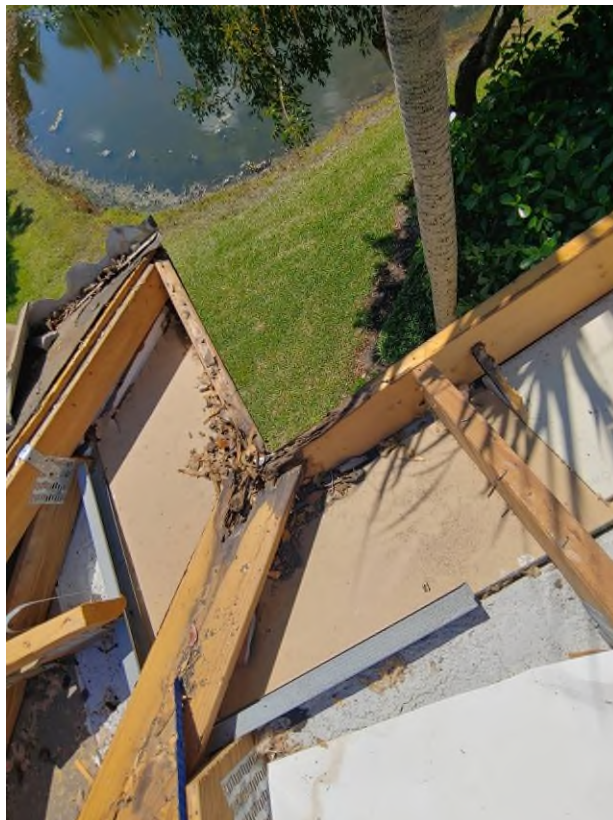
Photograph #12: Rotten fascia and trusses were observed on building 7890.
