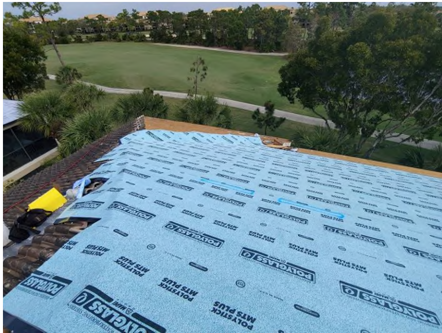
Photograph #9: Polystick MTS Plus underlayment installation was in progress on building 21751.
