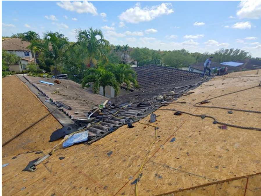
Photograph #13: Roof tile removal was in progress on building 21770.
