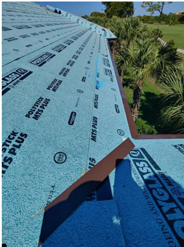
Photograph #18: Drip edge installation was in progress on building 21751.
