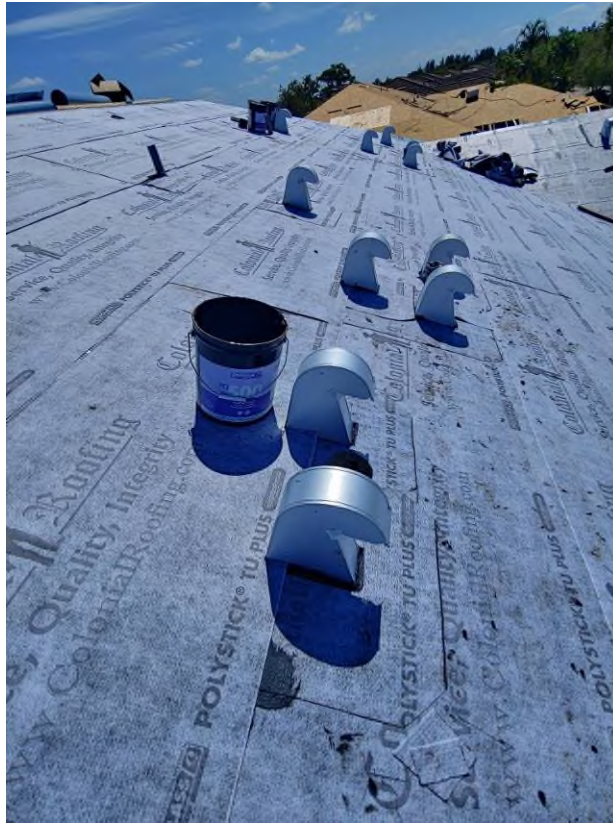
Photograph #17: Pipe and exhaust vent installations were in progress on building 21751.
