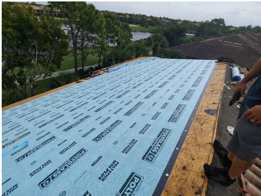
Photograph #10: Polystick MTS Plus underlayment installation was in progress on building 21751.
