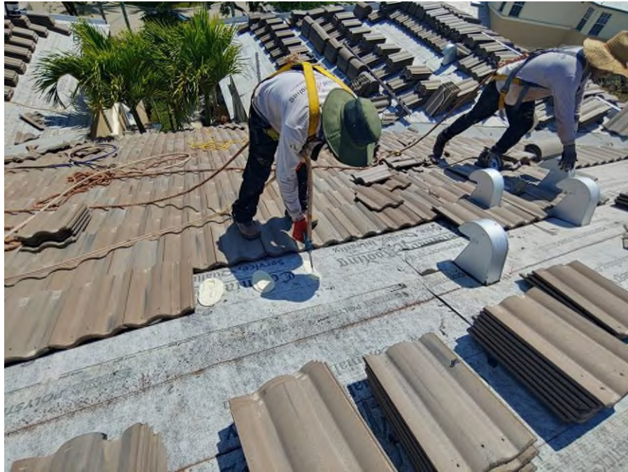
Photograph #5: Roof field tile installations with polyurethane foam adhesive was in progress on building 21700.
