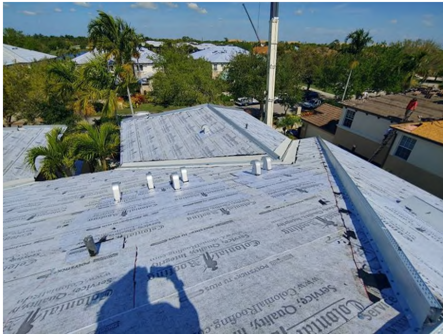
Photograph #1: Second layer of underlayment installation was completed on building 7880.
