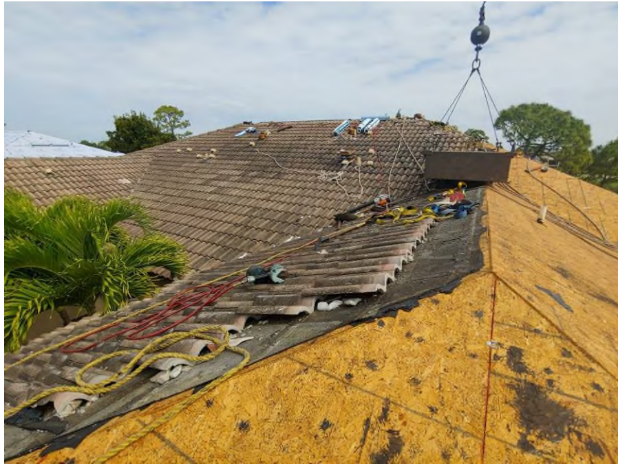
Photograph #5: Roof tile removal was in progress on building 21751.
