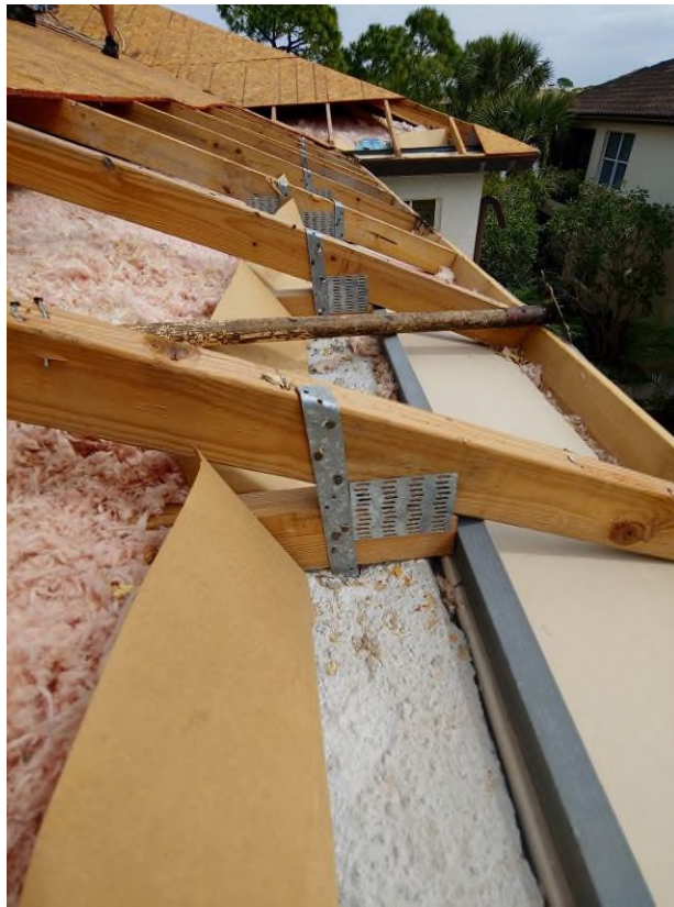
Photograph #7: Existing strap clips on the trusses have the required minimum quantity of nails on building 21751.
