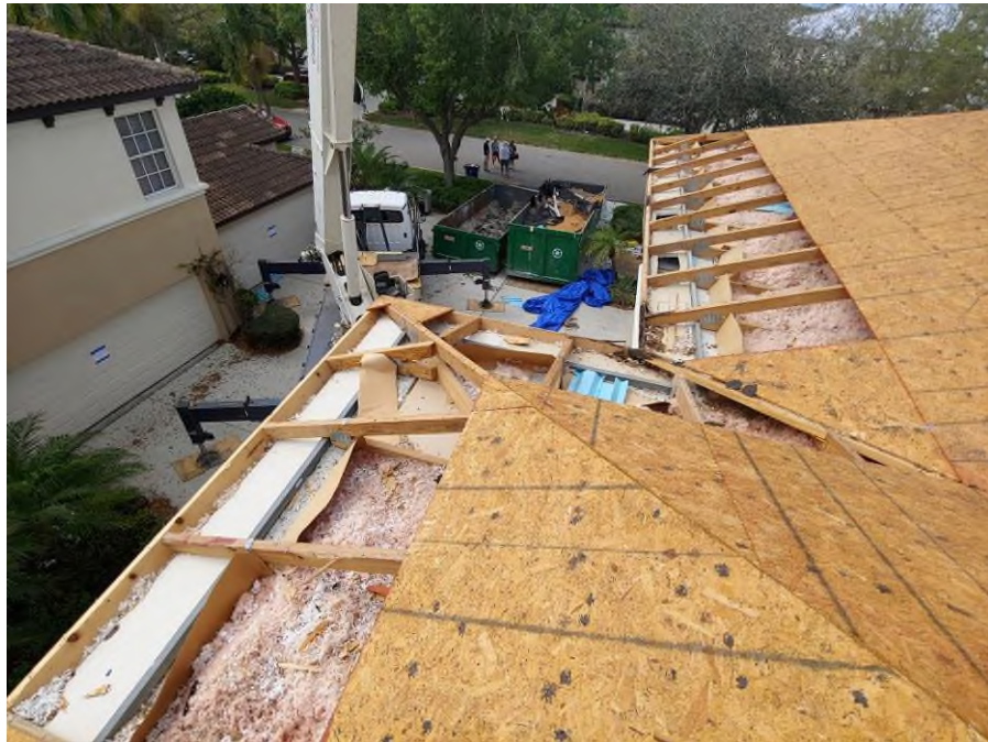
Photograph #6: Existing strap clips on the trusses have the required minimum quantity of nails on building 21751.
