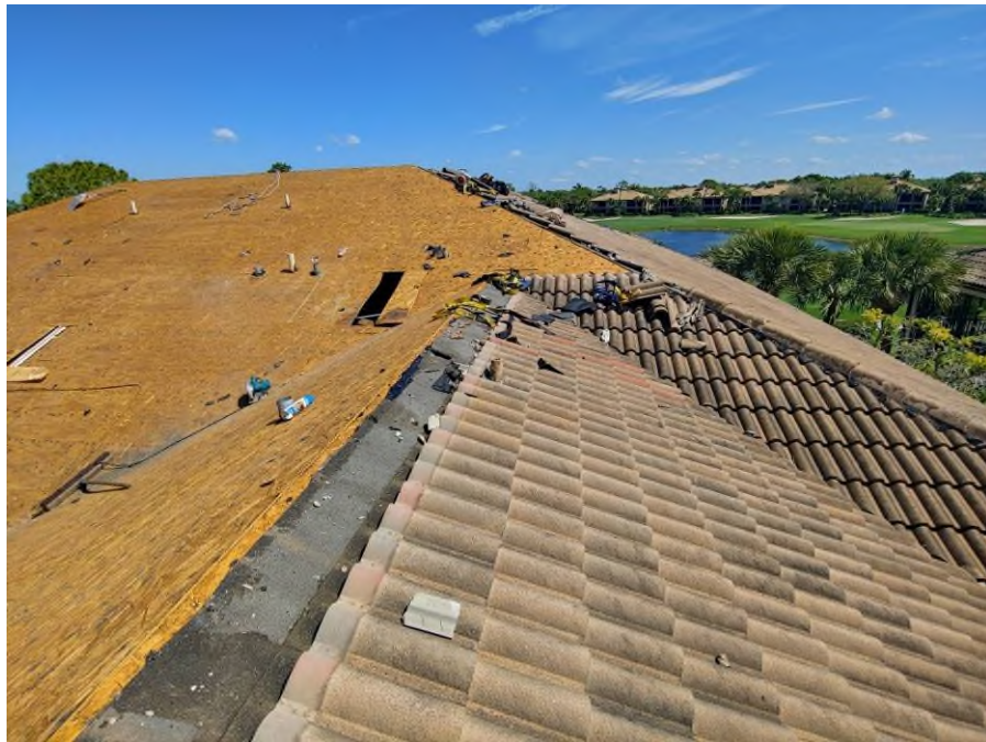
Photograph #22: Roof tile removal was in progress on building 21761.
