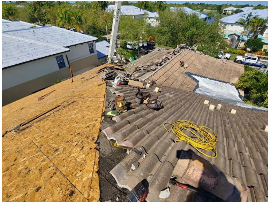
Photograph #9: Roof tile removal was in progress on building 7890.
