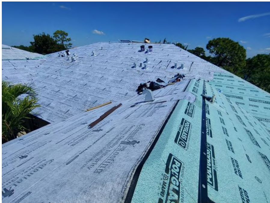
Photograph #16: Second layer of underlayment installation was in progress on building 21751.
