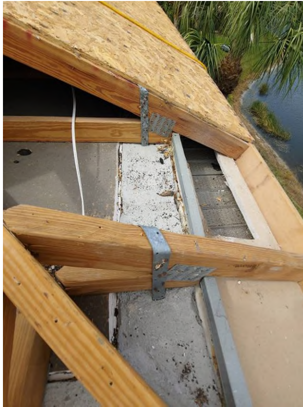
Photograph #3: Existing strap clips on the trusses have the required minimum quantity of nails on building 7881.
