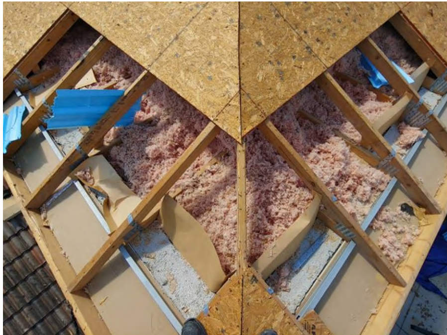
Photograph #14: Existing strap clips on the trusses have the required minimum quantity of nails on building 21770.
