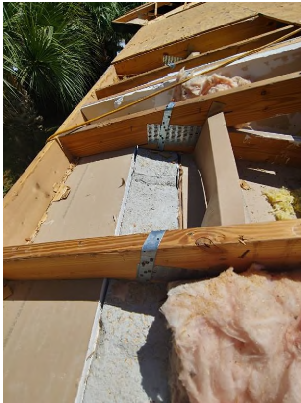
Photograph #12: Existing strap clips on the trusses have the required minimum of 5 nails on building 21841.
