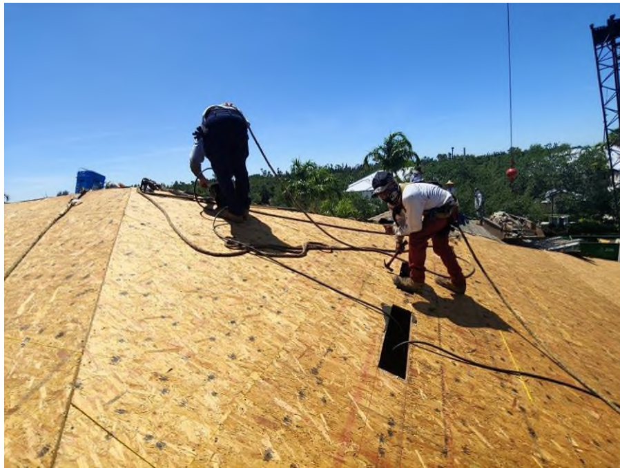
Photograph #15: Re-nail pattern at the plywood sheathing was in progress on building 21841.
