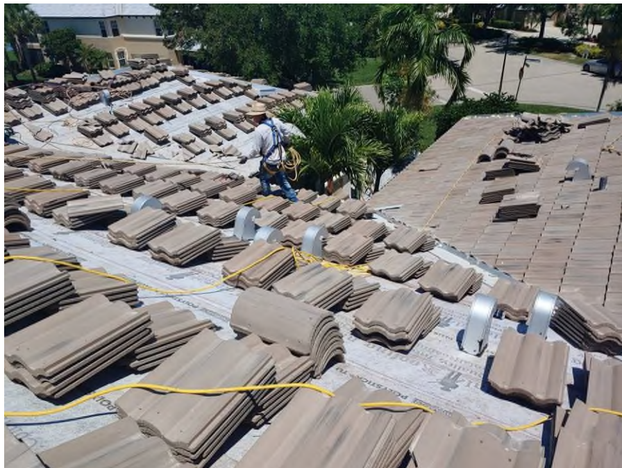
Photograph #2: Roof field tile installation with polyurethane foam adhesive was in progress on building 21800.
