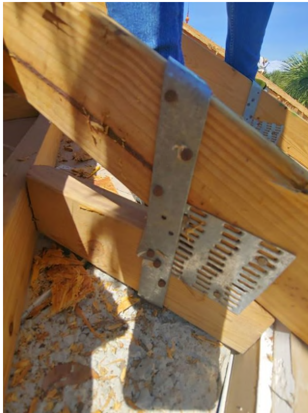
Photograph #6: Existing strap clips on the trusses have the required minimum of 5 nails on building 21831.
