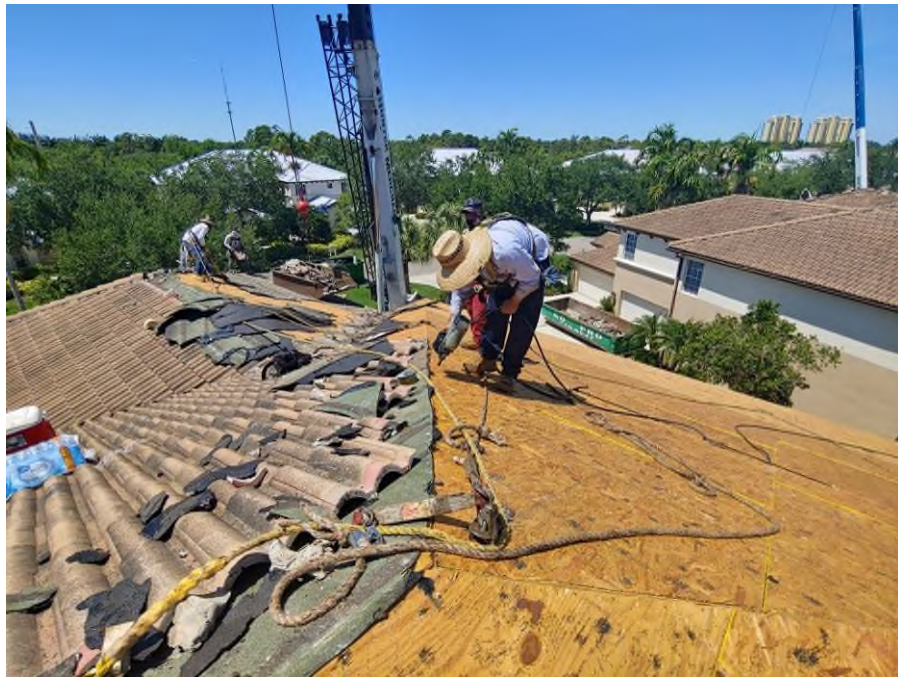
Photograph #11: Re-nail pattern at the plywood sheathing was in progress on building 21841.
