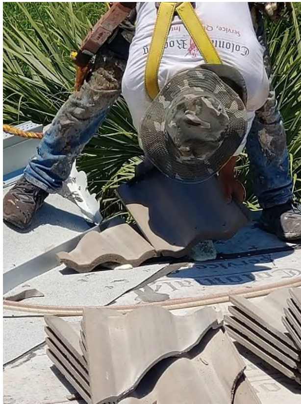
Photograph #3: Roof field tile installation with polyurethane foam adhesive was in progress on building 21800.
