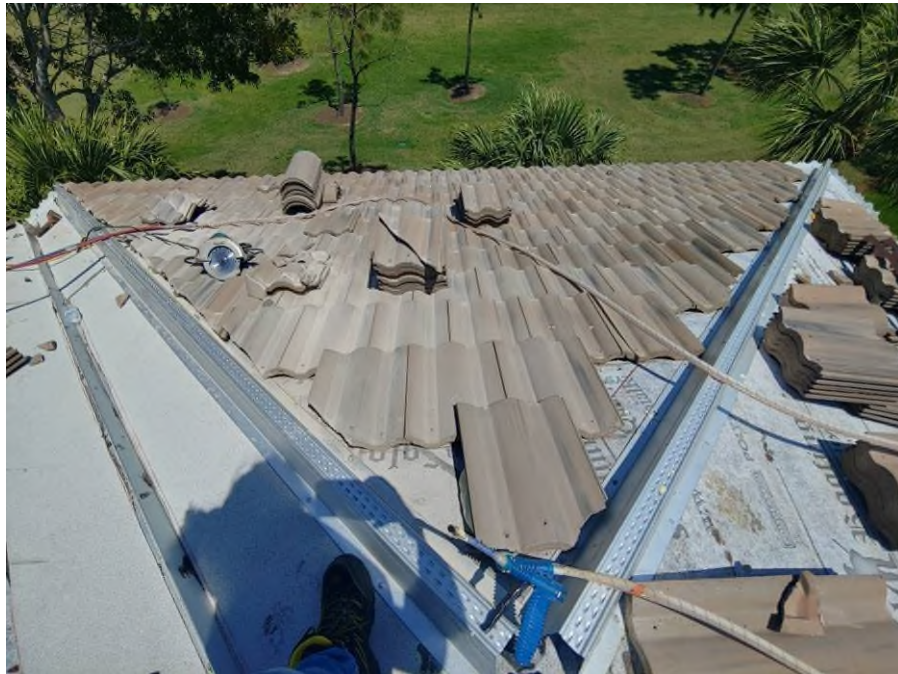
Photograph #10: Roof field, ridge and hip tile installations with polyurethane foam adhesive were in progress on building 21721.
