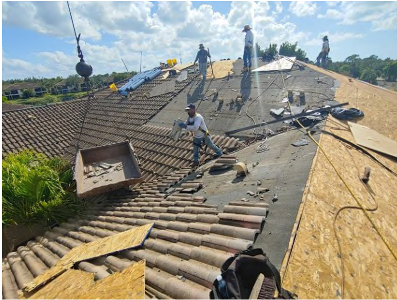
Photograph #17: Roof tile removal was in progress on building 21710.
