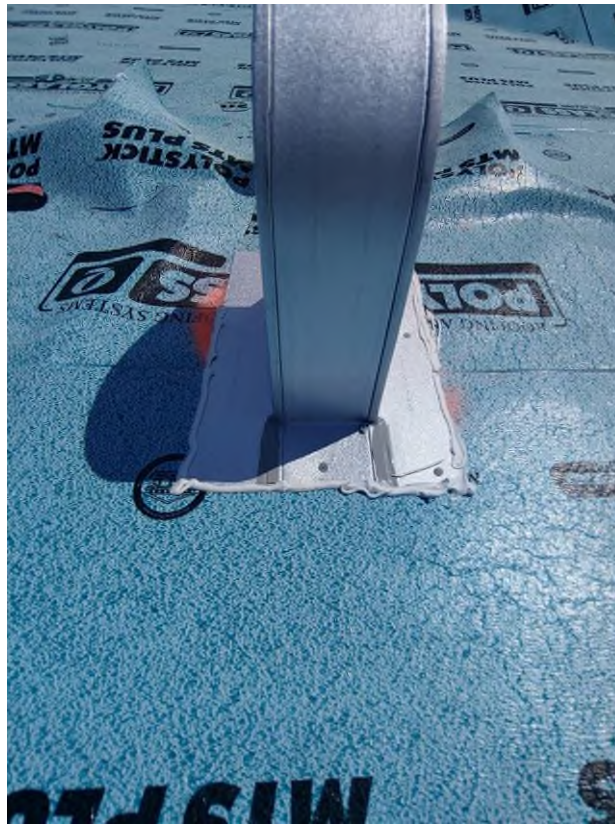
Photograph #23: Exhaust vent installations were in progress on building 21711.
