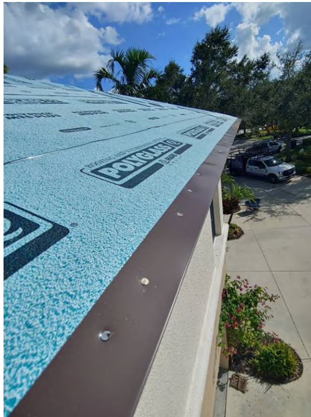
Photograph #21: Drip-edge flashing installation was completed on building 21711.
