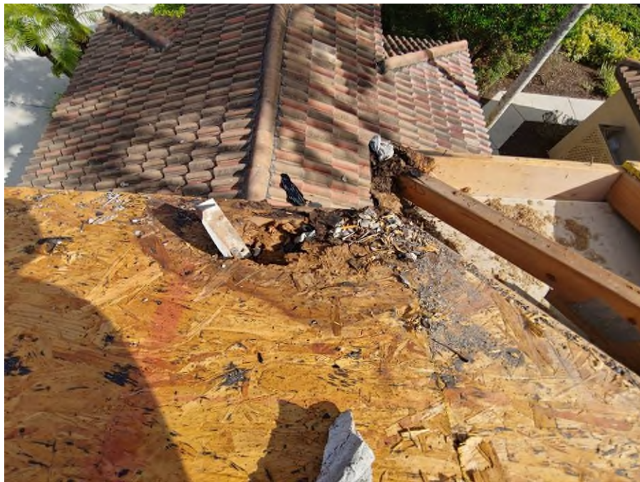
Photograph #8: Rotten plywood sheathing was observed on building 7841.
