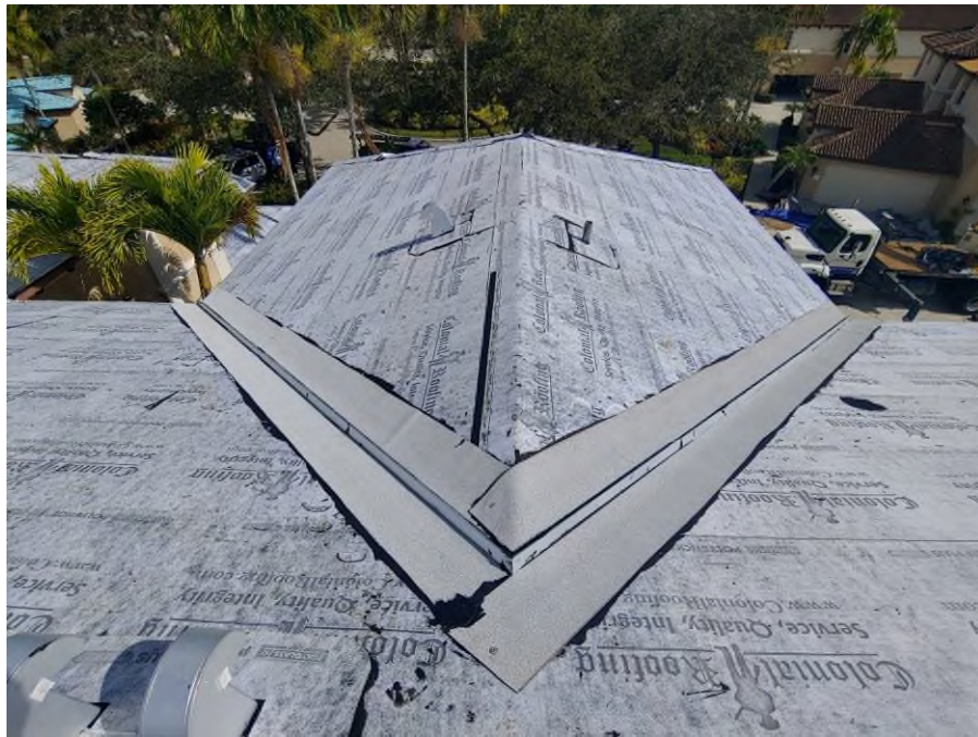
Photograph #15: Valley installations were in progress on buildings 21700.
