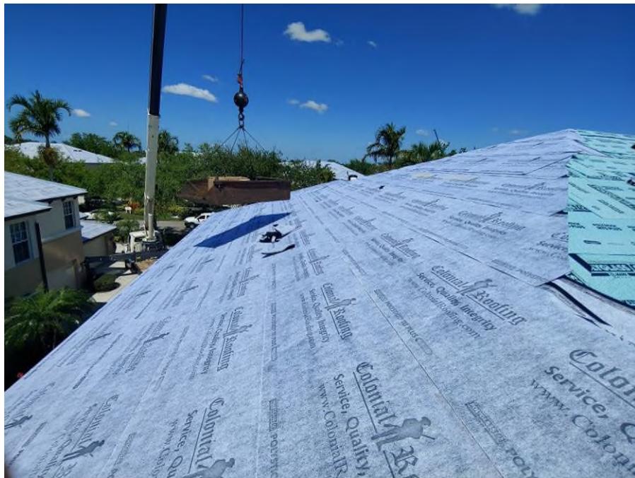
Photograph #12: Second layer of underlayment installation was in progress on building 7890.
