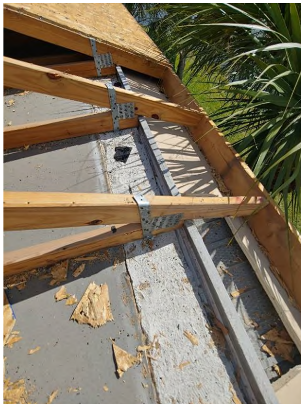
Photograph #18: Existing strap clips on trusses have the required minimum quantity of nails on building 21710
