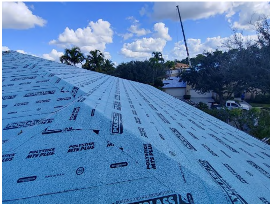
Photograph #10: Underlayment installation was in progress on the west side of buildings 7841.
