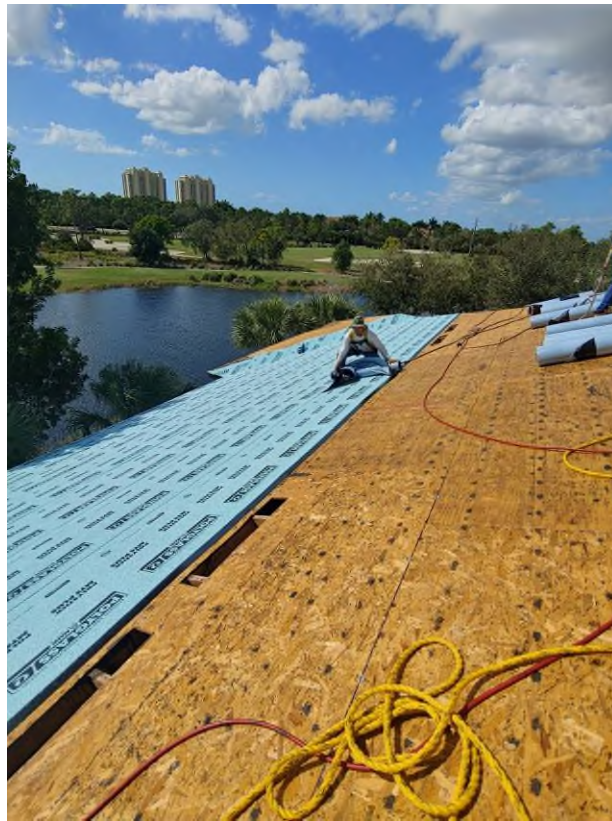
Photograph #19: Underlayment installation was in progress on the west side of buildings 21710.
