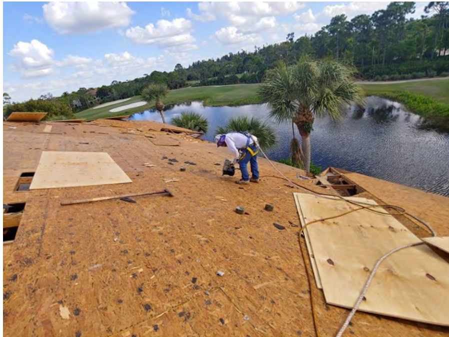
Photograph #14: Re-nail pattern at plywood sheathing was in progress on building 7850.
