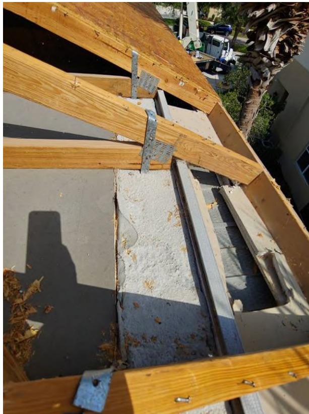
Photograph #18: Existing strap clips on trusses have the required minimum quantity of nails on building 21720.
