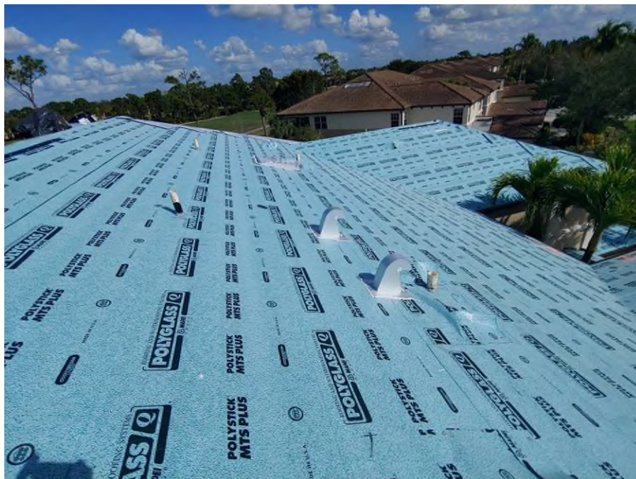
Photograph #22: Exhaust vent installations were in progress on building 21711.
