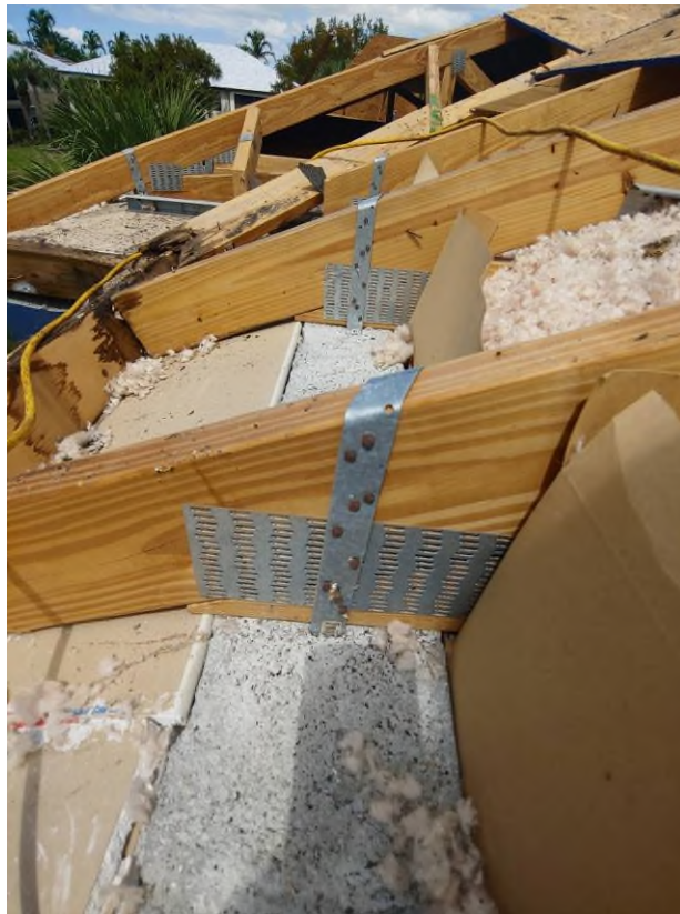
Photograph #27: Existing strap clips on the trusses have the required minimum of nails on building 21820.
