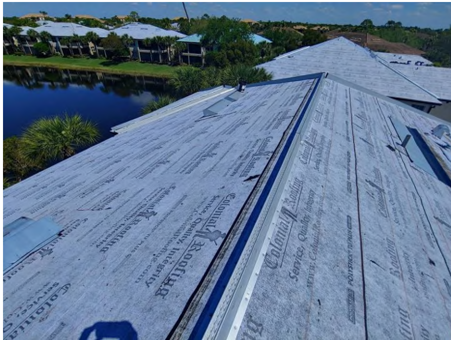
Photograph #7: Second layer of underlayment installation was completed on building 7881.
