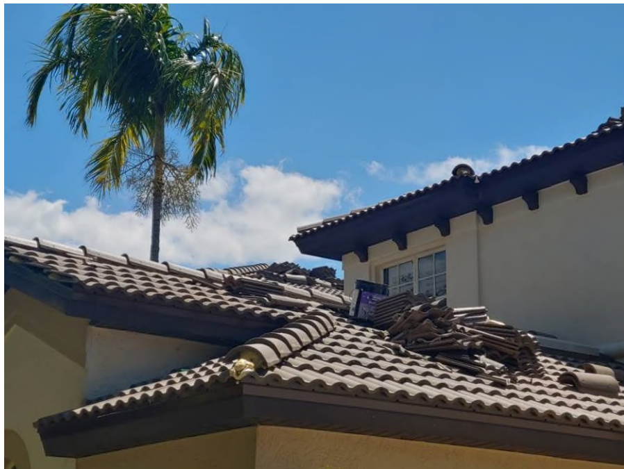
Photograph #2: Roof field, ridge and hip tile installations with polyurethane foam adhesive were in progress on building 21710.
