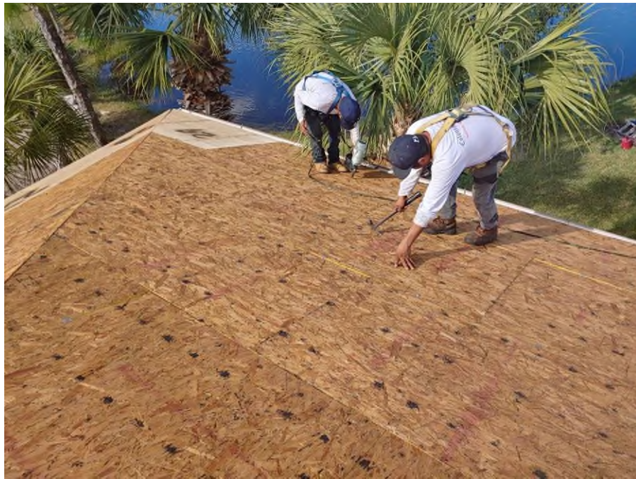
Photograph #7: Re-nail pattern at plywood sheathing was in progress on building 7841.
