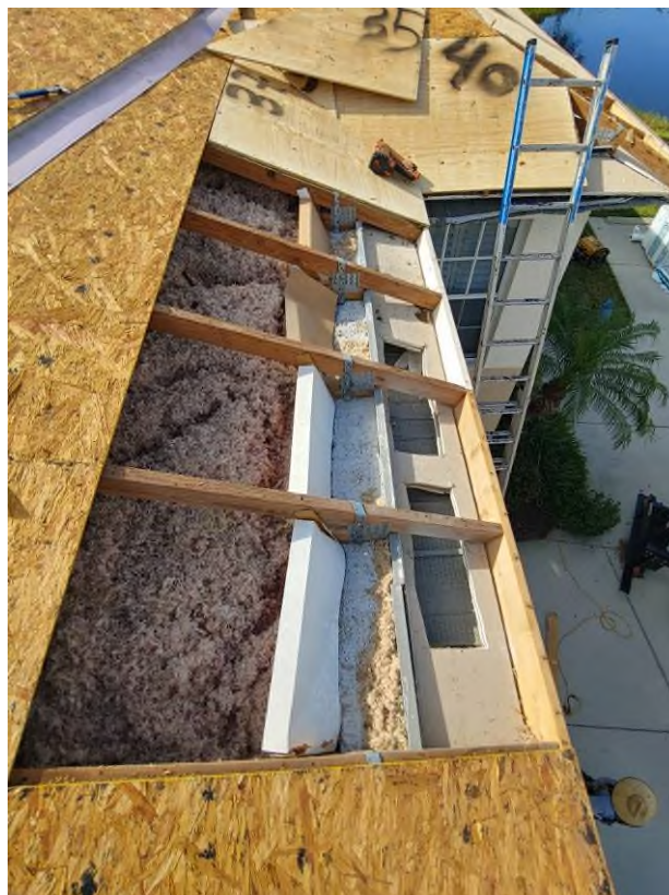
Photograph #6: Existing strap clips on trusses have the required minimum quantity of nails on building 7841.
