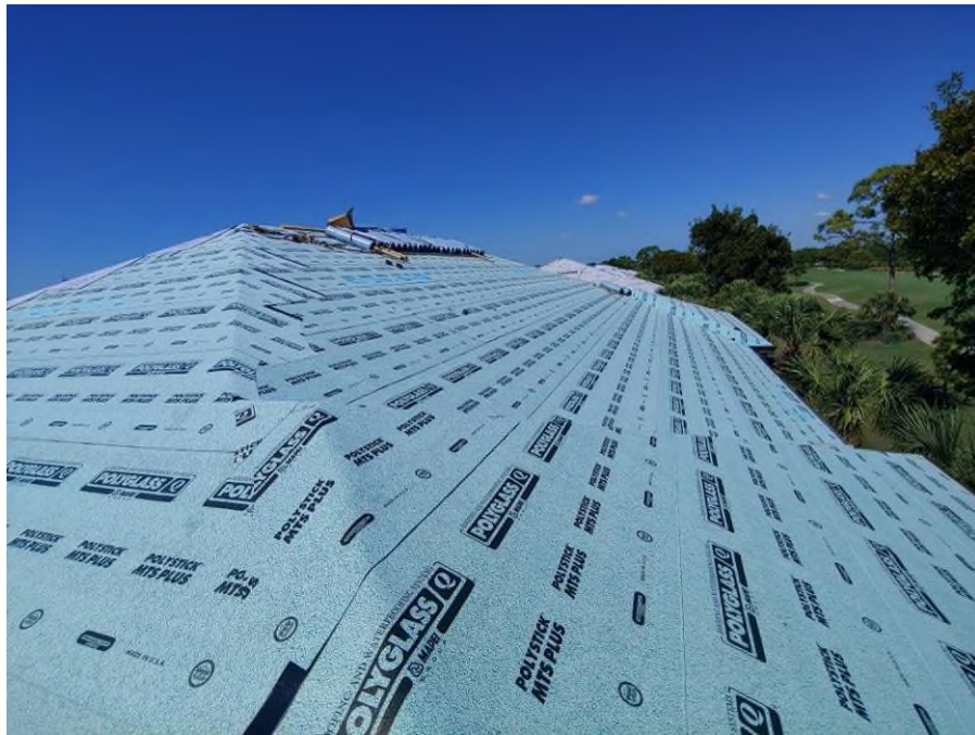
Photograph #15: Polystick MTS Plus underlayment installation was completed on building 21751.
