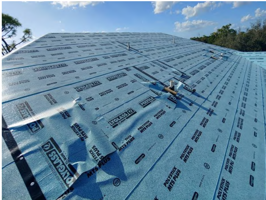
Photograph #4: Exhaust vent installations were in progress on building 7840.
