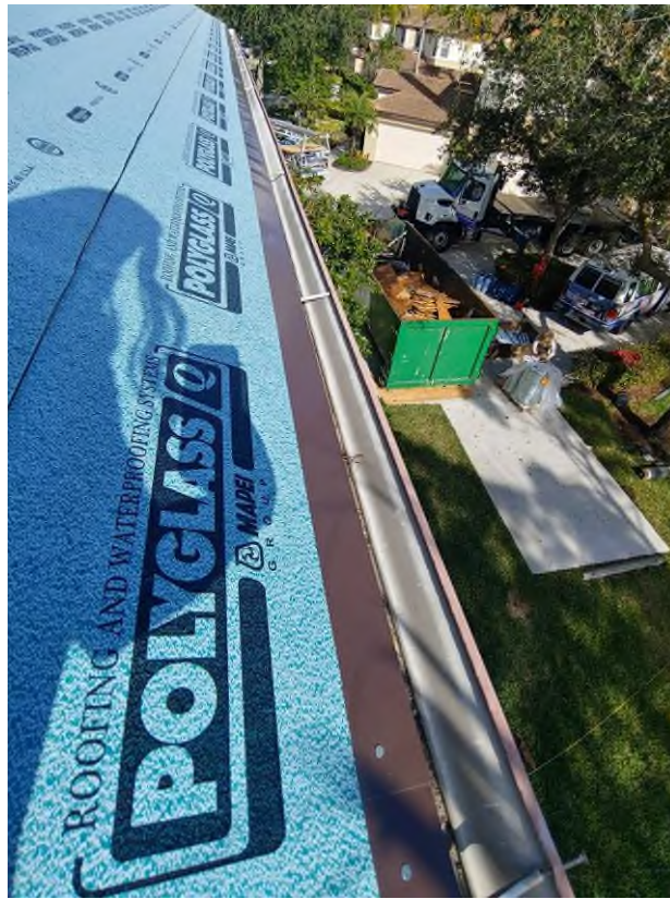
Photograph #3: Drip-edge flashing installation was in progress on building 7840.
