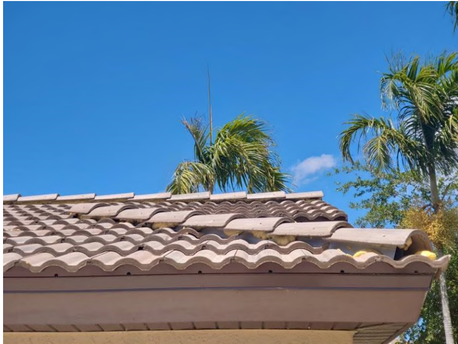
Photograph #1: Roof field, ridge and hip tile installations with polyurethane foam adhesive were in progress on building 21710.
