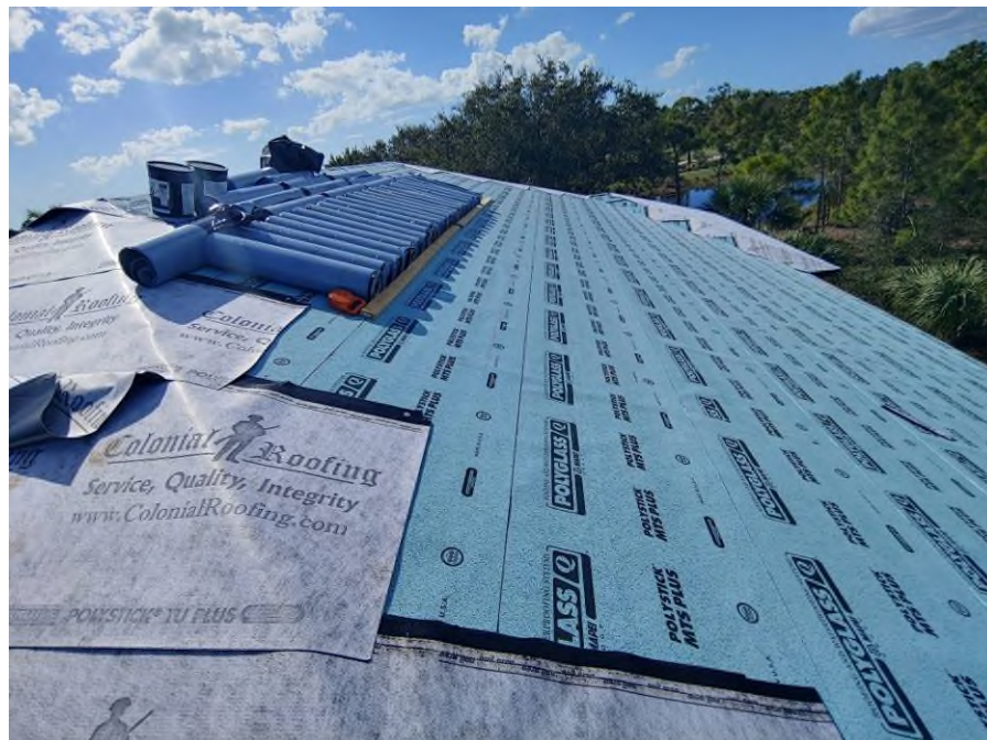
Photograph #20: Polystick MTS Plus underlayment was completed and second layer of underlayment was in progress on building 21711.
