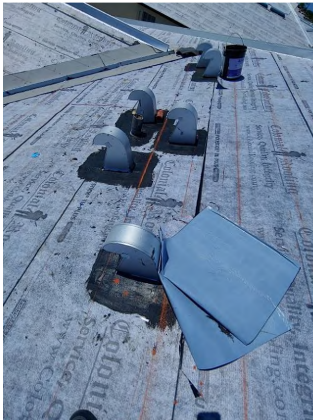
Photograph #10: Pipe and exhaust vent installations were in progress on building 7881.
