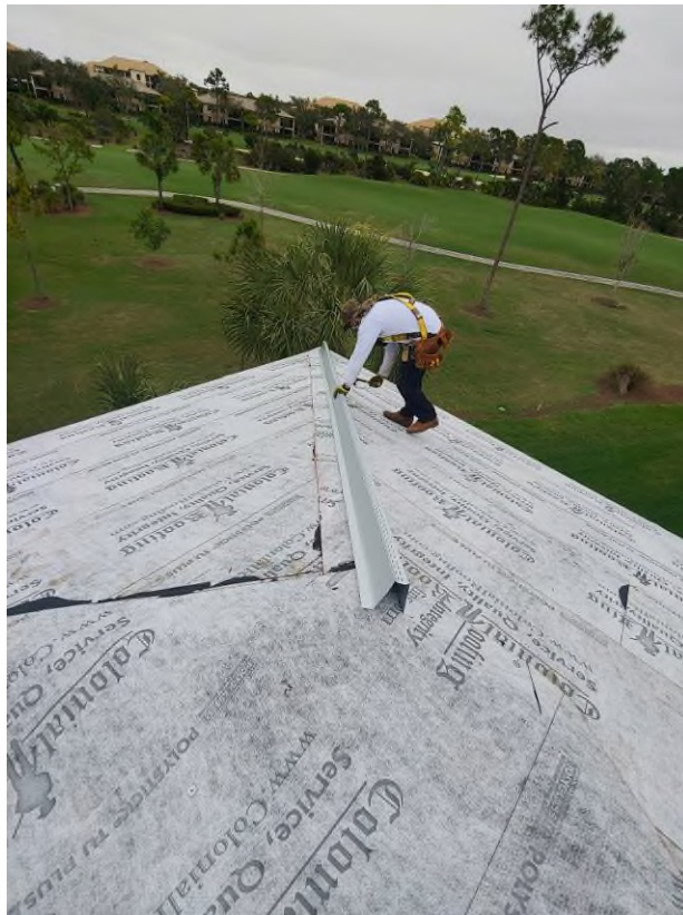
Photograph #12: V-crimp metal valley flashing, and hip/ridge metal channel installations were in progress on building 21711.
