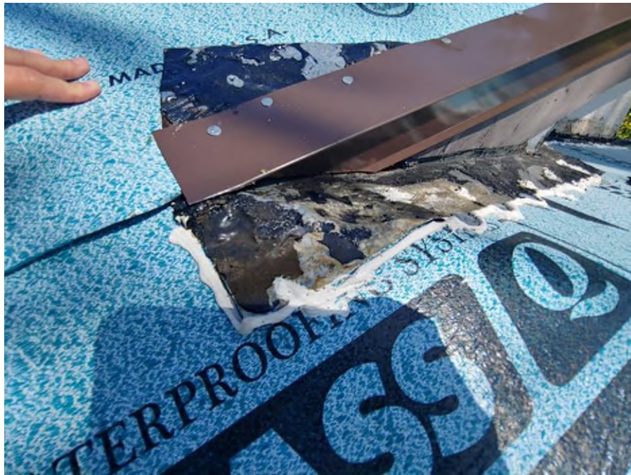
Photograph #9: Contractor must address sealant application on the metal flashing on building 7841.
