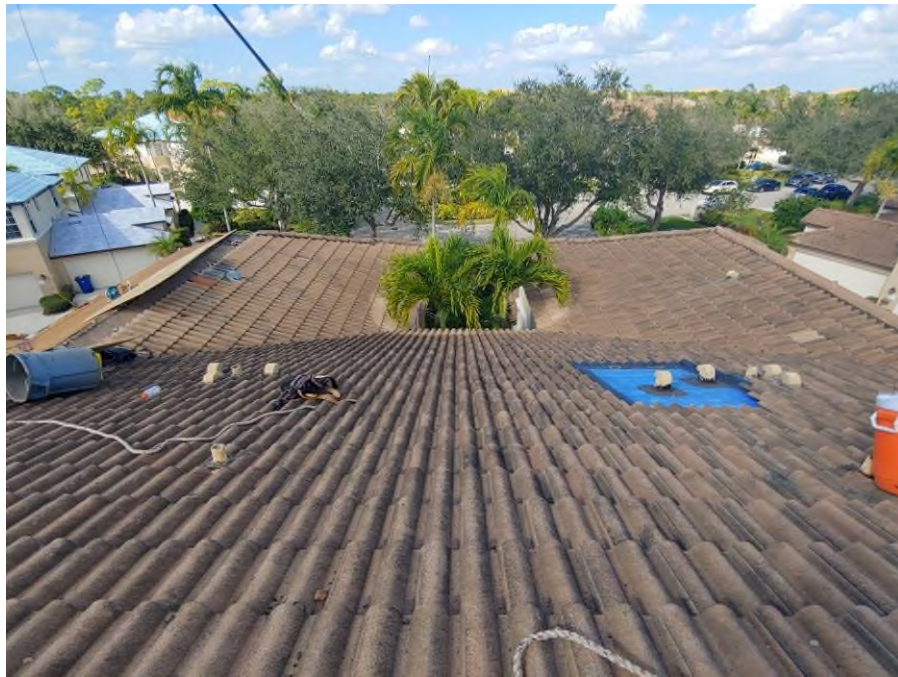
Photograph #11: Roof tile removal was in progress on building 7850.
