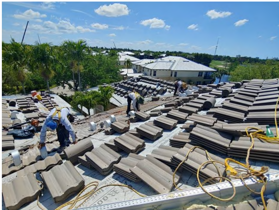
Photograph #4: Roof field tile installations with polyurethane foam adhesive was in progress on building 21700.
