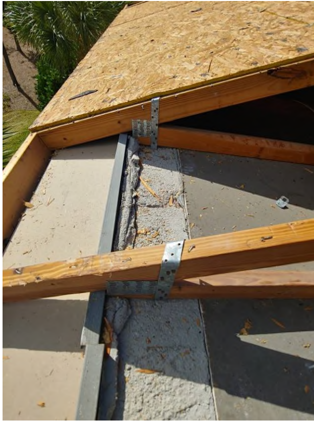
Photograph #13: Existing strap clips on trusses have the required minimum quantity of nails on building 7850.
