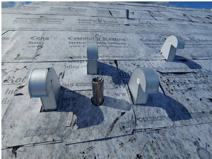
Photograph #16: Exhaust vent installations were completed on building 21700.
