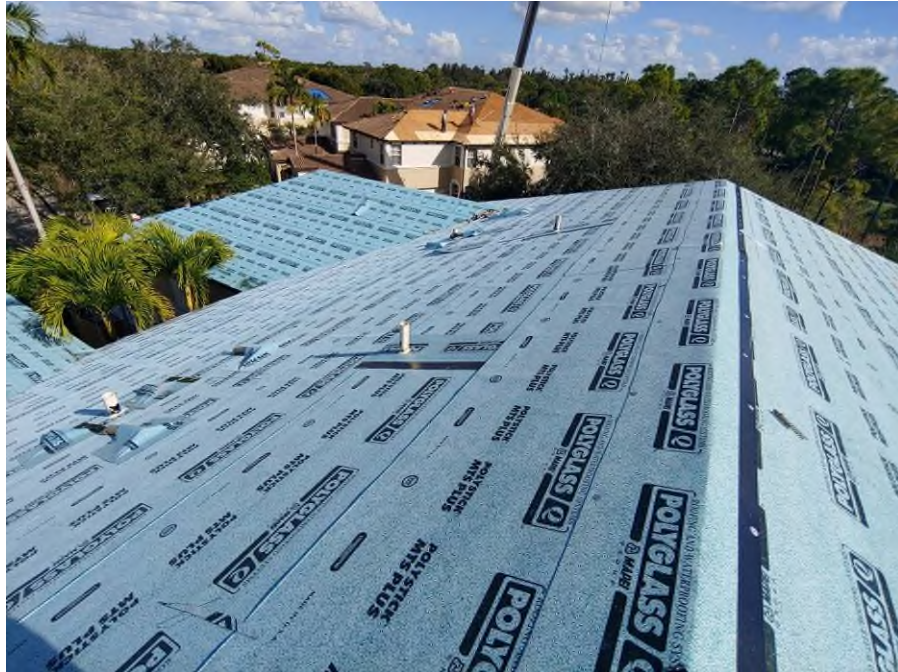
Photograph #1: Polystick MTS Plus underlayment was completed on building 7840.
