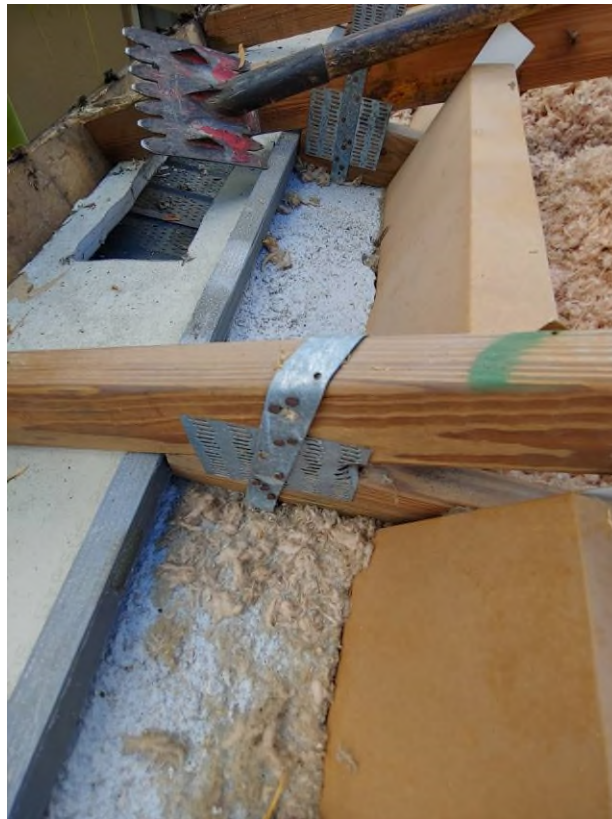
Photograph #5: Existing strap clips on trusses have the required minimum quantity of nails on building 7841.
