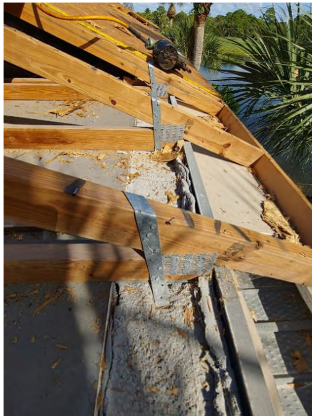
Photograph #12: Existing strap clips on trusses have the required minimum quantity of nails on building 7850.
