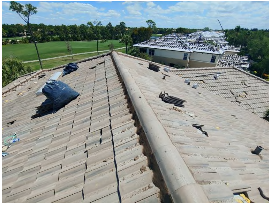
Photograph #5: Roof field, ridge and hip tile installations with polyurethane foam adhesive were in progress on building 21711.
