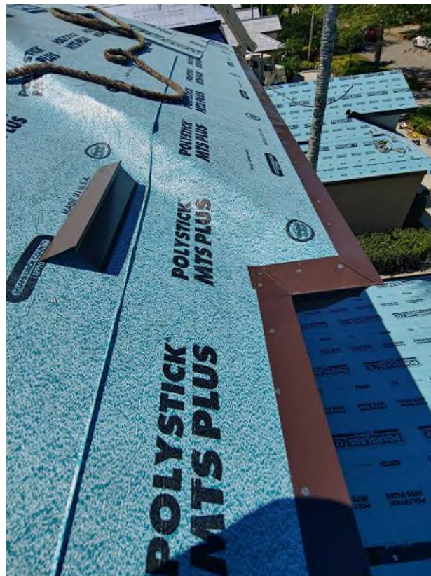
Photograph #14: Drip edge installation was in progress on building 7890.
