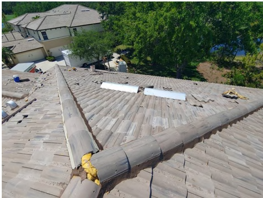
Photograph #6: Roof field, ridge and hip tile installations with polyurethane foam adhesive were in progress on building 21711.
