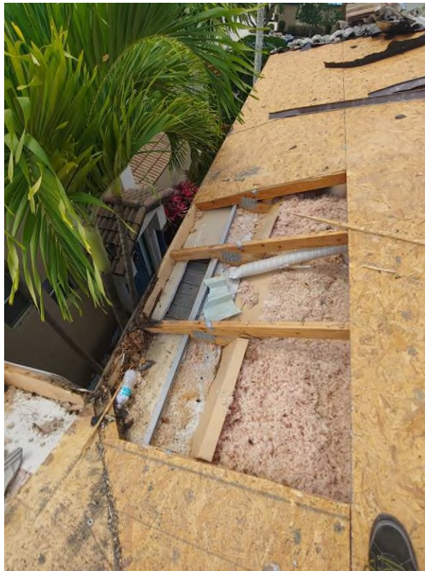
Photograph #10: Existing strap clips on the trusses have the required minimum quantity of nails on building 21771.
