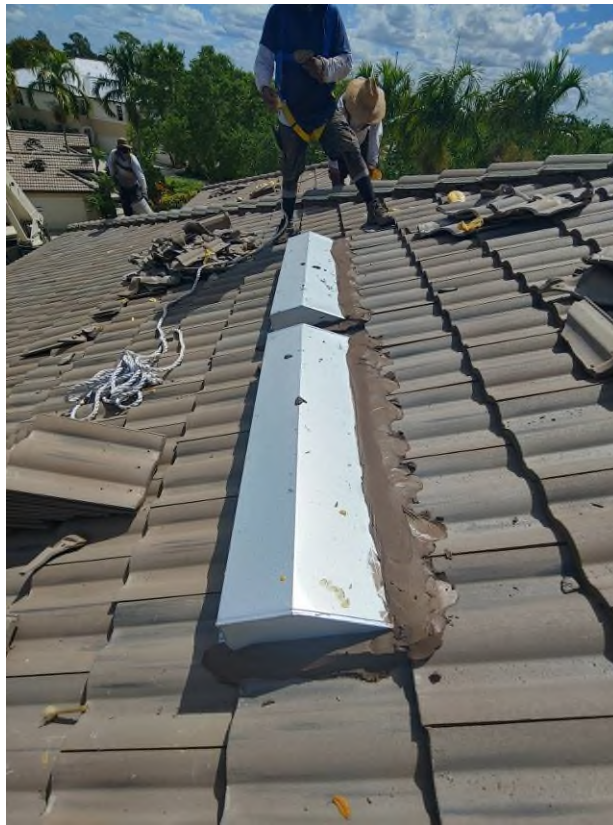
Photograph #3: Mortar adhesive application was in progress surrounding the exhaust vents on building 21700.
