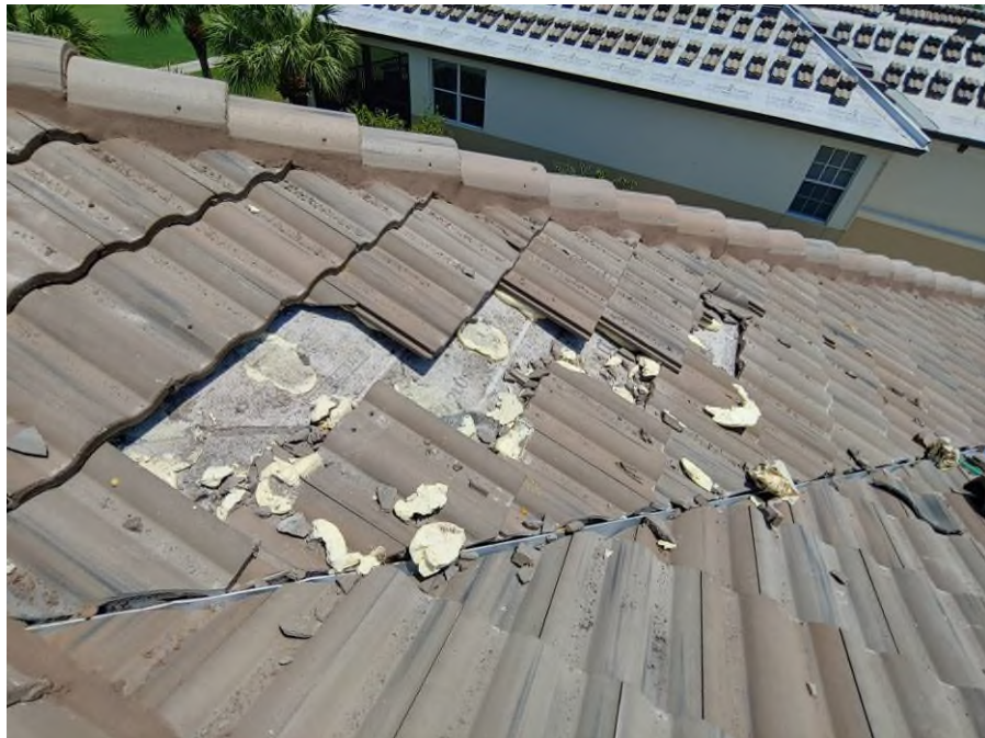
Photograph #4: Broken field tile replacement was in progress on building 21731.
