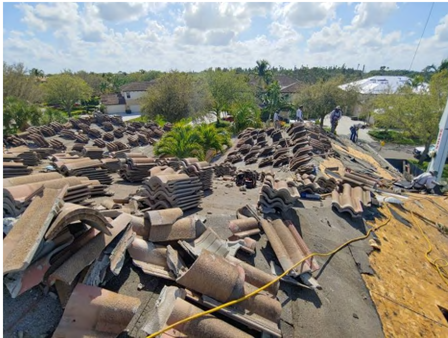
Photograph #1: Roof tile removal was in progress on building 7891.
