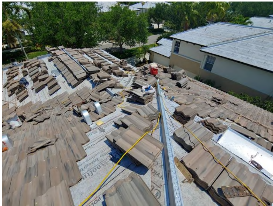
Photograph #8: Roof field tiles with polyurethane foam adhesive were in progress on building 21760.
