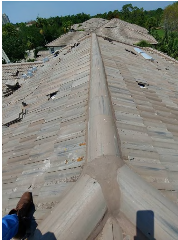
Photograph #1: Mortar adhesive application was in progress on building 21731.
