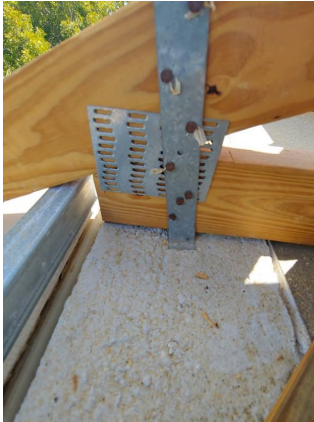
Photograph #3: Existing strap clips on the trusses have the required minimum of nails on building 7891.
