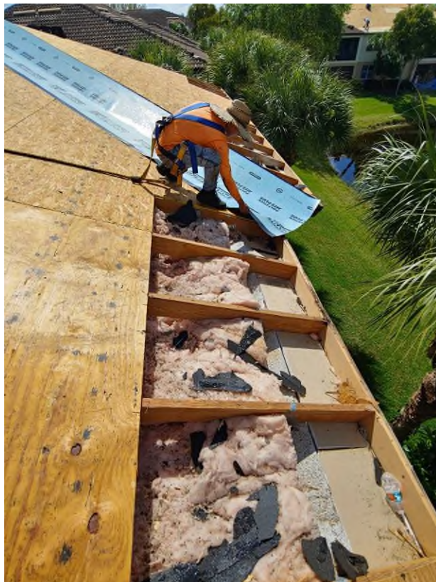
Photograph #8: Polystick MTS underlayment installation was in progress on building 21760.
