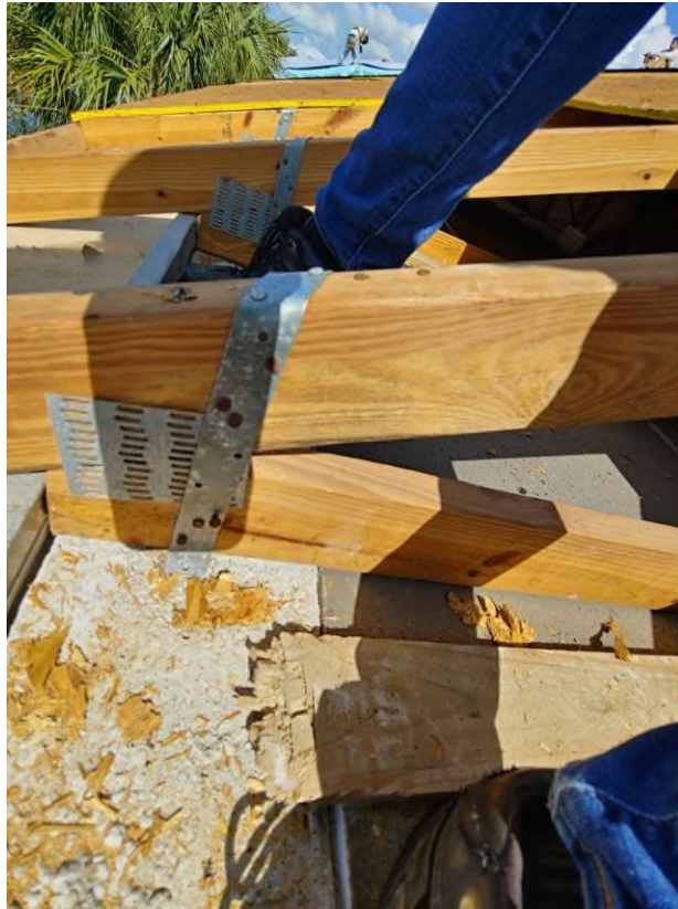
Photograph #7: Existing strap clips on the trusses have the required minimum of nails on building 21760.
