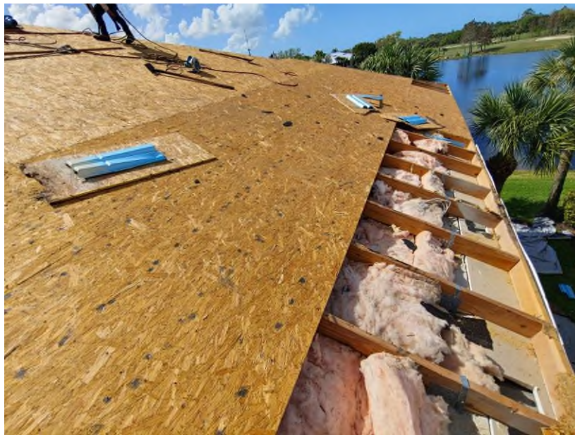
Photograph #6: Existing strap clips on the trusses have the required minimum of nails on building 21760.
