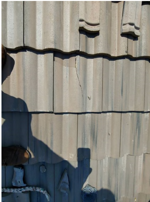
Photograph #9: Broken field tile replacement must be addressed on building 21760.
