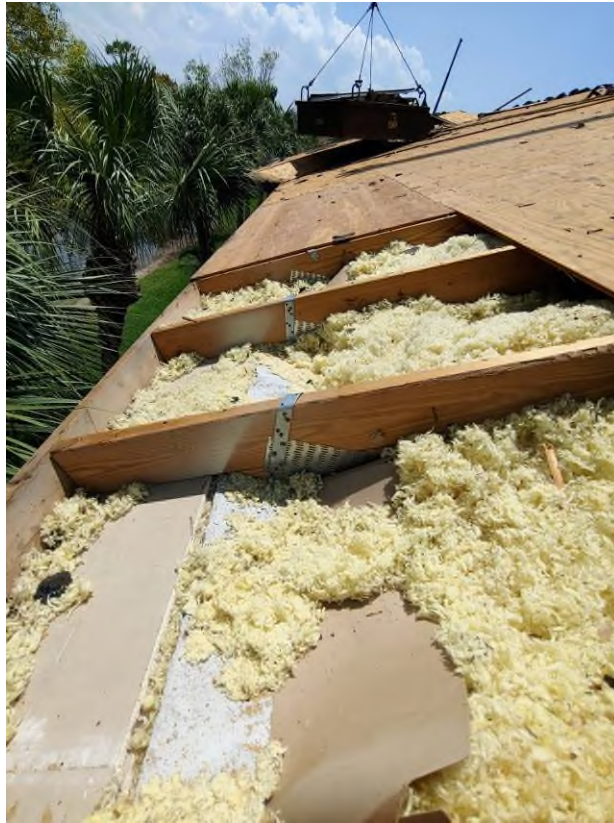
Photograph #13: Existing strap clips on the trusses have the required minimum of 5 nails on building 21811.
