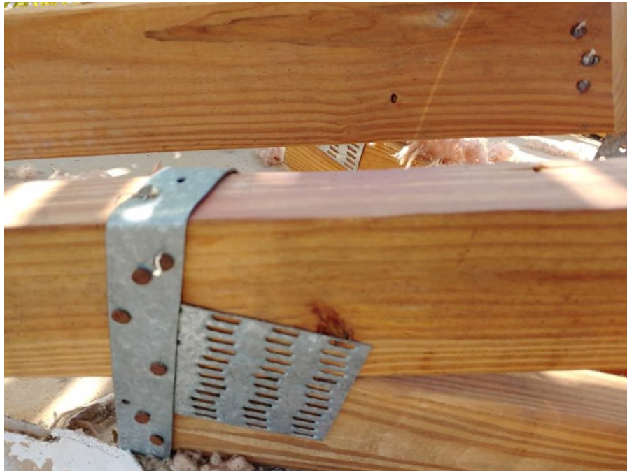
Photograph #4: Existing strap clips on the trusses have the required minimum of nails on building 7891.
