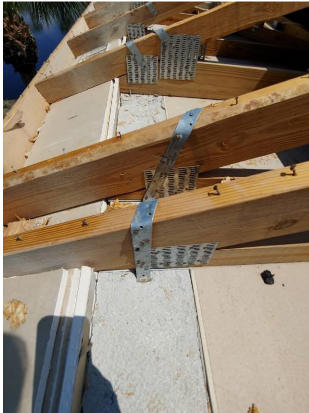
Photograph #14: Existing strap clips on the trusses have the required minimum of 5 nails on building 21811.
