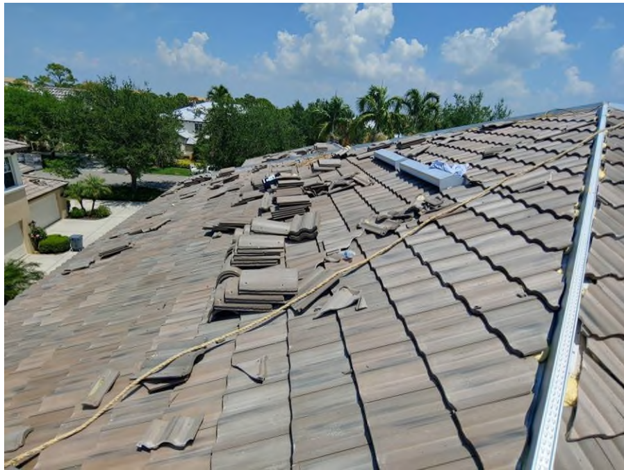
Photograph #7: Roof field tiles with polyurethane foam adhesive were in progress on building 21760.
