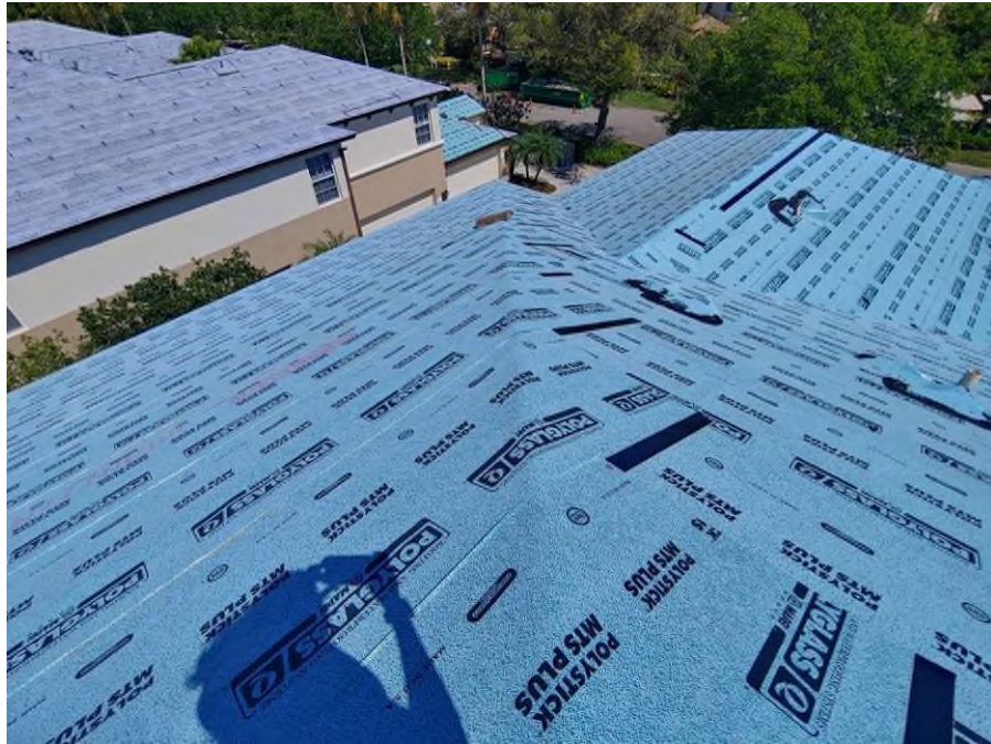
Photograph #19: Polystick MTS Plus underlayment installation was completed on building 21770.
