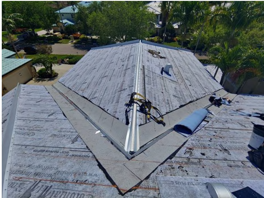
Photograph #8: V-crimp metal valley flashing installations were in progress on building 7881.
