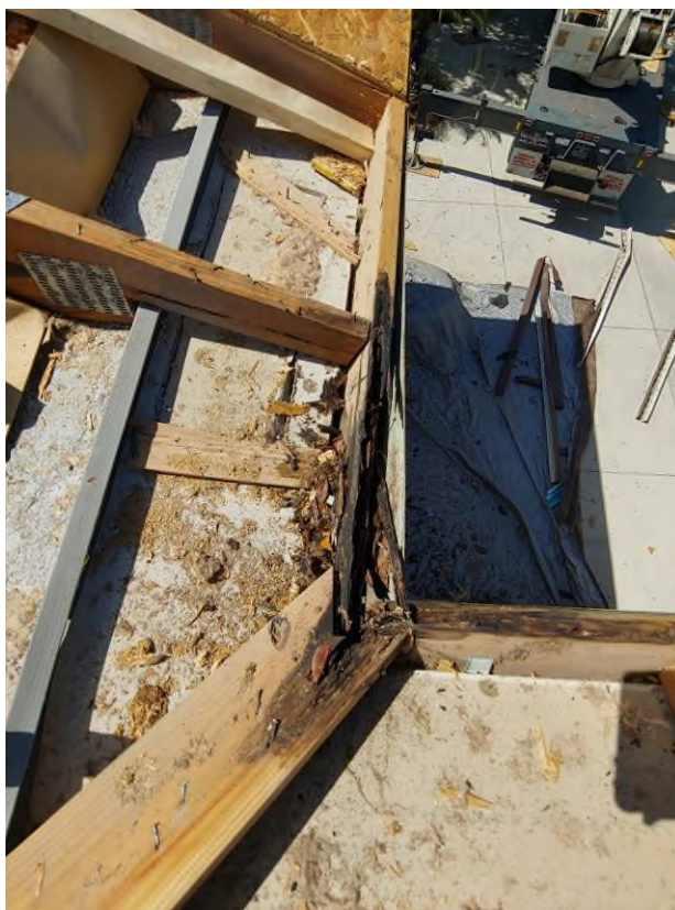
Photograph #25: Rotten fascia and trusses were observed on building 21761.
