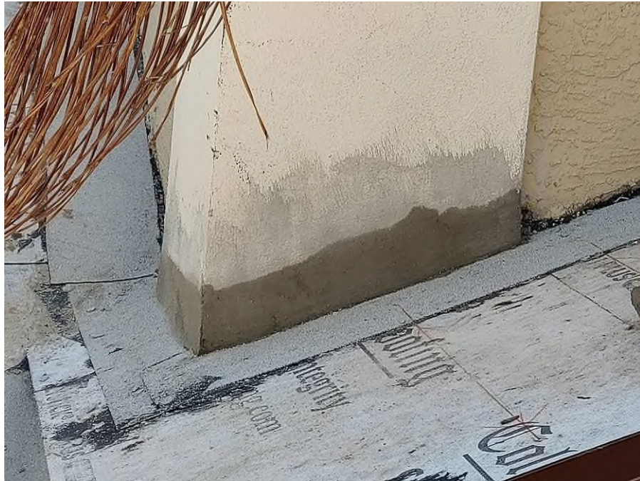
Photograph #3: Stucco application was completed on the columns at building 7840.
