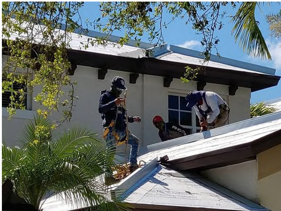
Photograph #8: Hip/ridge metal channel installation was in progress on building 7881.
