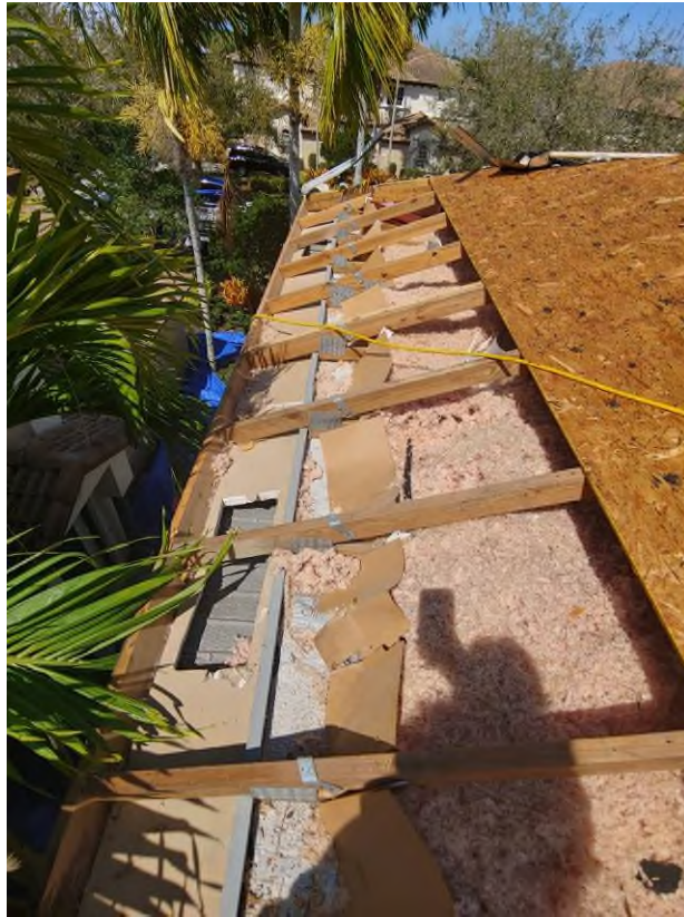
Photography #5: Existing strap clips on the trusses have the required minimum quantity of nails on building 7880.
