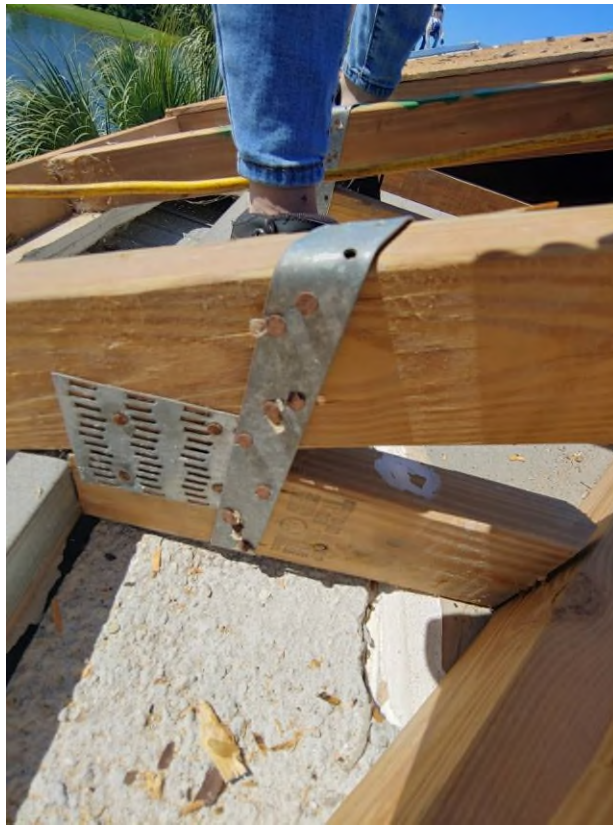
Photograph #11: Existing strap clips on the trusses have the required minimum quantity of nails on building 7890.
