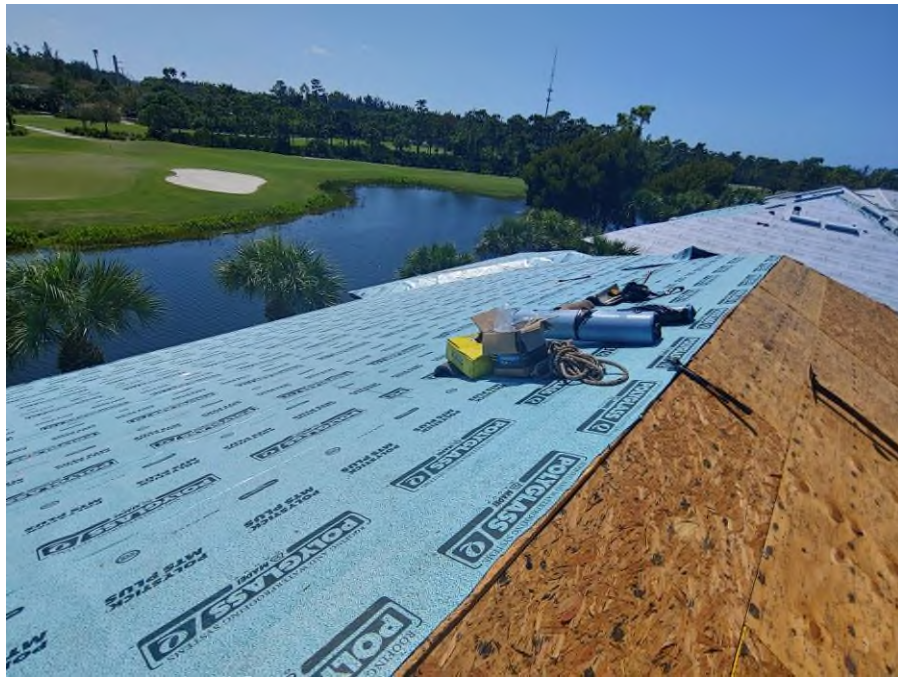
Photography #7: Polystick MTS Plus underlayment installation was in progress on building 7880.
