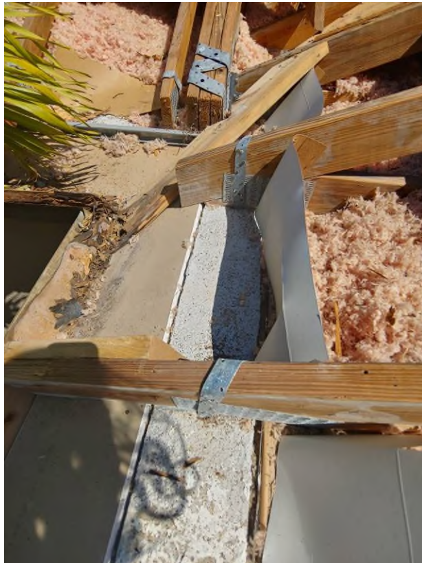
Photography #6: Existing strap clips on the trusses have the required minimum quantity of nails on building 7880.
