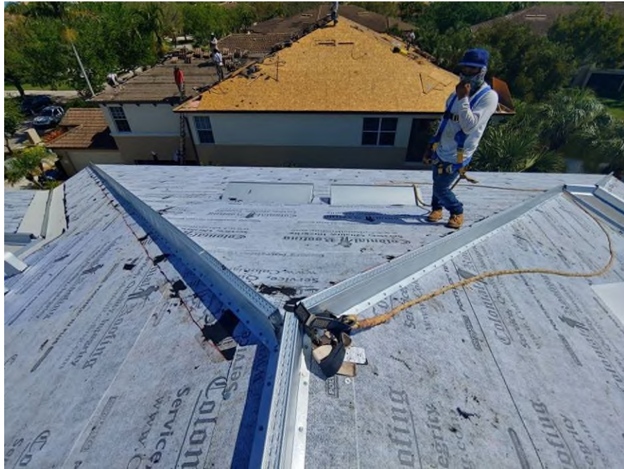
Photograph #5: Hip/ridge metal channel installation was in progress on building 7880.
