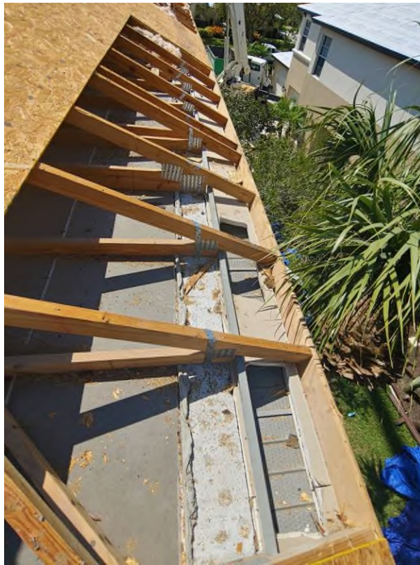
Photography #11: Existing strap clips on the trusses have the required minimum quantity of nails on building 21741.
