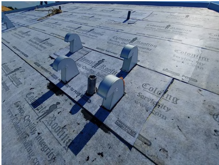
Photograph #2: Pipe and exhaust vent installations were completed on building 7880.
