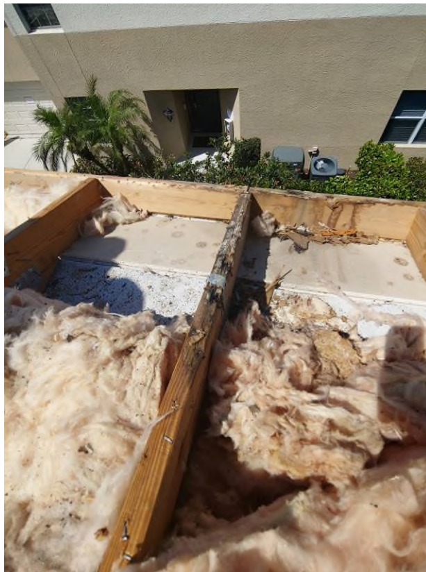
Photography #14: Rotten fascia and truss were observed on building 21741.
