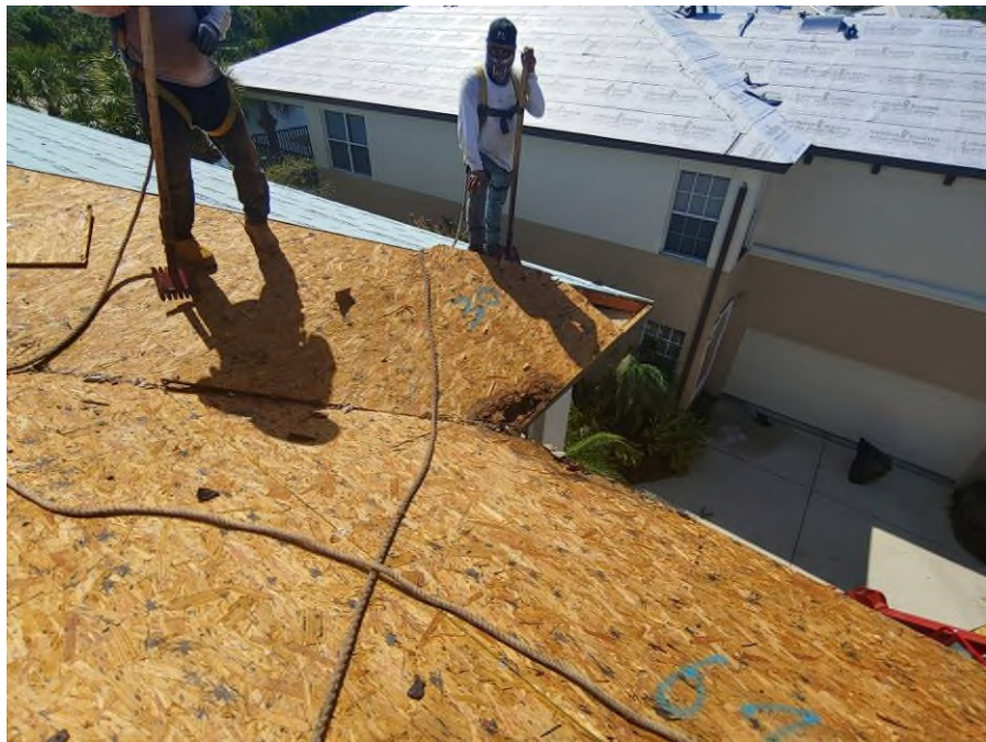
Photography #8: Rotten plywood sheathing was observed on building 7880.
