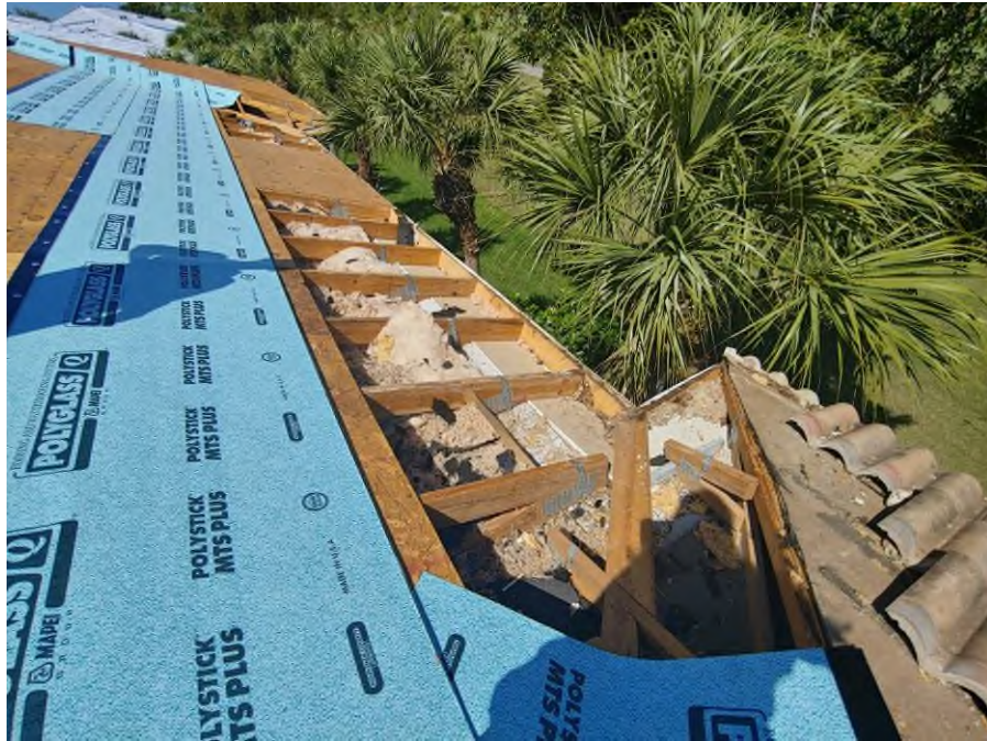
Photography #13: Polystick MTS Plus underlayment installation was in progress on building 21741.
