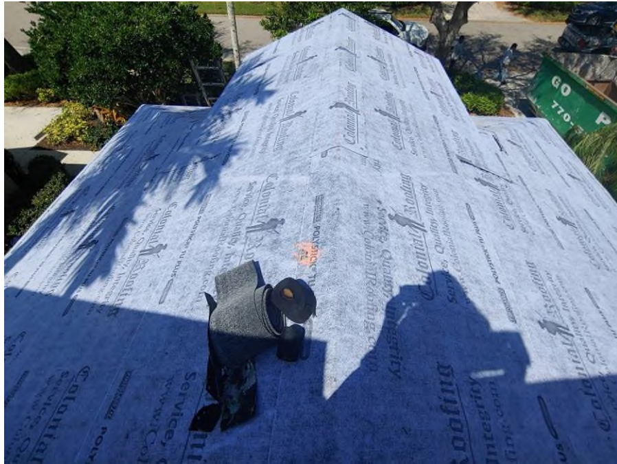
Photography #3: Second layer of underlayment installation was in progress on building 7870.
