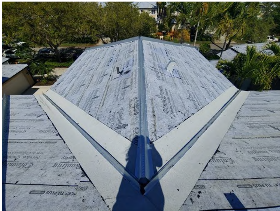
Photograph #4: V-crimp metal valley flashing installations were completed on building 7880.
