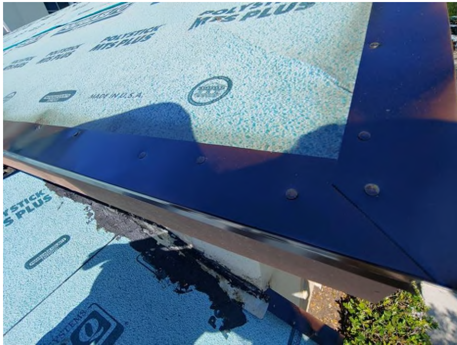
Photograph #5: Drip-edge flashing installation was in progress on the garage roof on building 21820.
