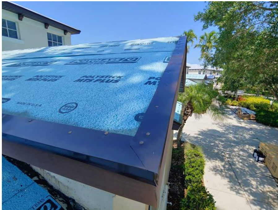
Photograph #5: Drip edge flashing installation was completed on building 21830.
