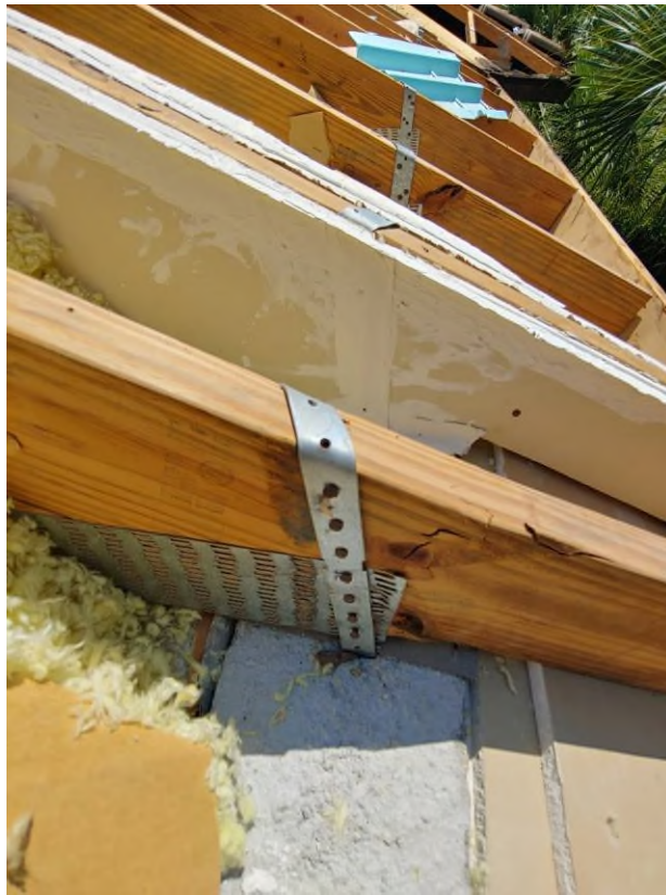
Photograph #9: Existing strap clips on the trusses have the required minimum quantity of 5 nails on building 21840.
