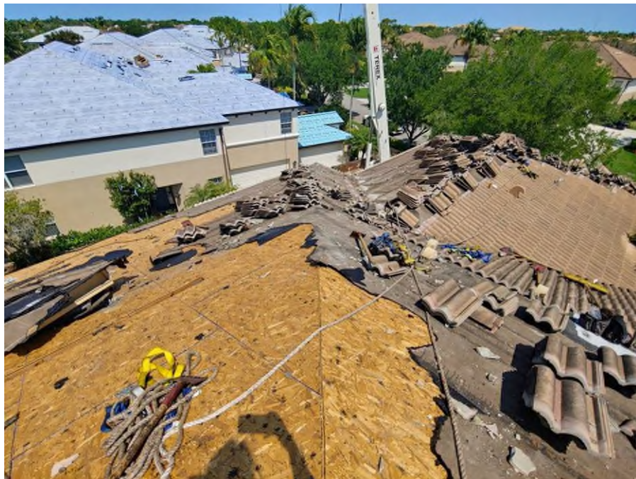
Photograph #6: Roof tile removal was in progress on building 21840.
