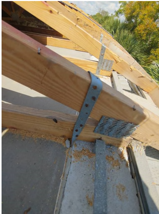
Photograph #3: Existing strap clips on the trusses have the required minimum of 5 nails on building 21791.
