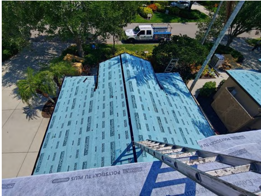
Photograph #1: Polystick MTS Plus underlayment installation was completed on building 21830.
