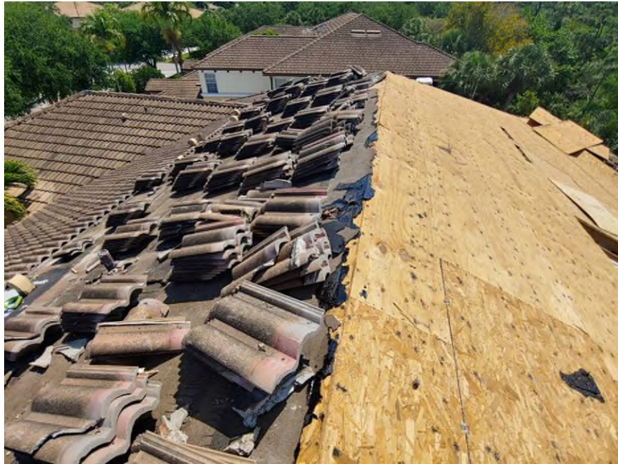
Photograph #7: Roof tile removal was in progress on building 21840.
