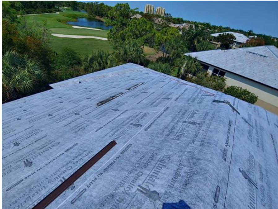
Photograph #3: Second layer of underlayment installation was in progress on building 21830.
