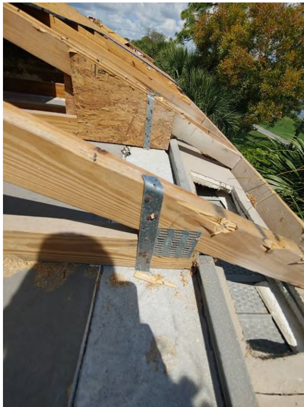
Photograph #4: Existing strap clips on the trusses have the required minimum of 5 nails on building 21791.
