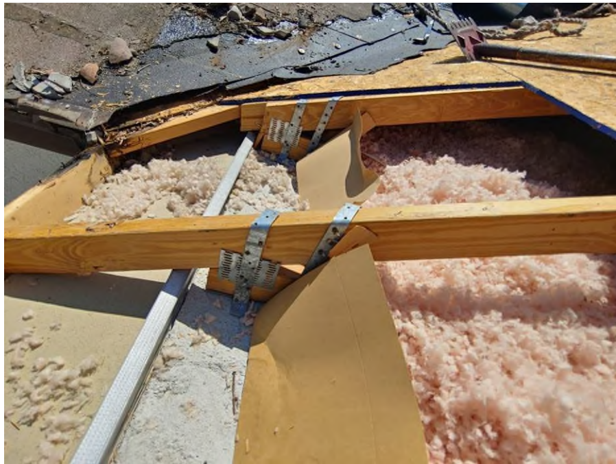
Photograph #9: Existing strap clips on the trusses have the required minimum quantity of 5 nails on building 21830.
