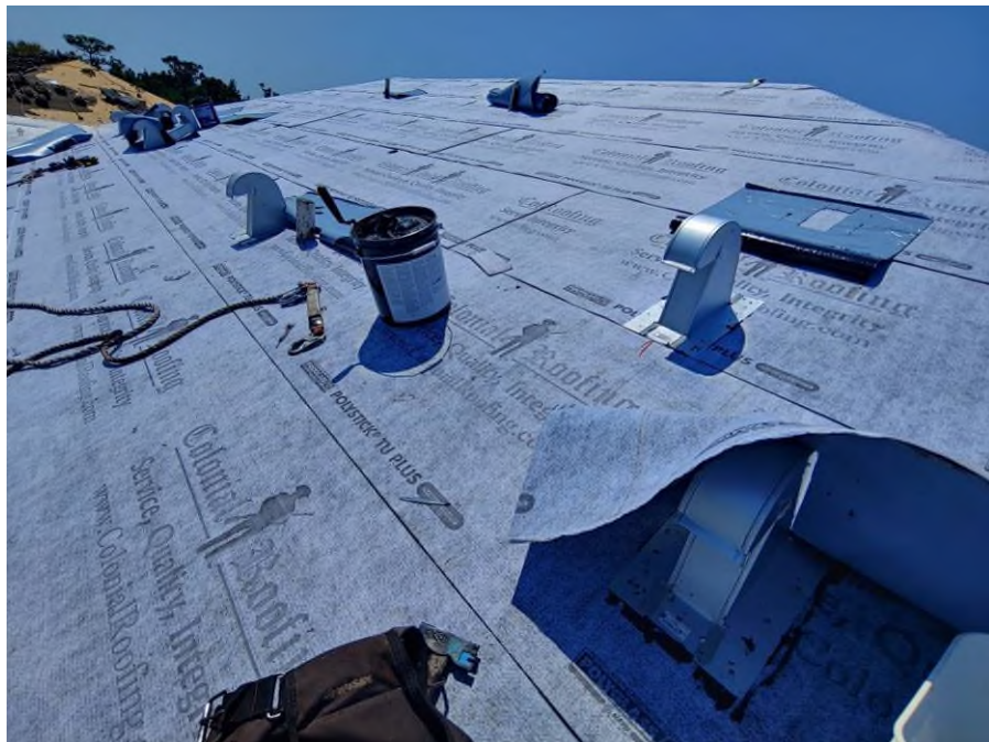
Photograph #4: Exhaust vent installations were in progress on building 21830.
