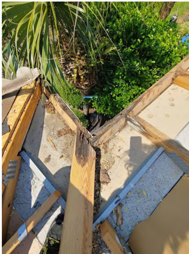
Photograph #10: Rotten fascia, truss and plywood sheathing were observed building 21840.
