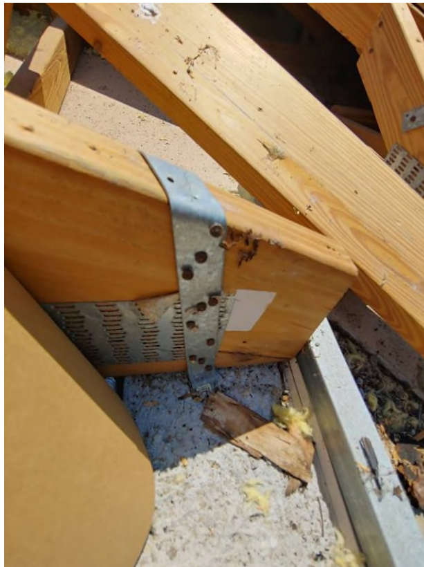
Photograph #8: Existing strap clips on the trusses have the required minimum quantity of 5 nails on building 21840.
