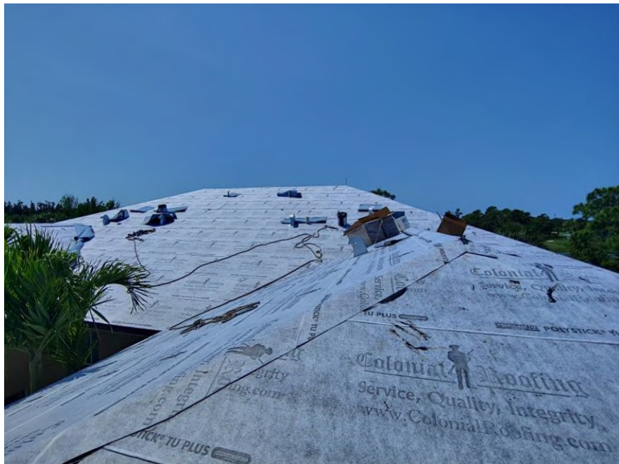
Photograph #2: Second layer of underlayment installation was in progress on building 21830.
