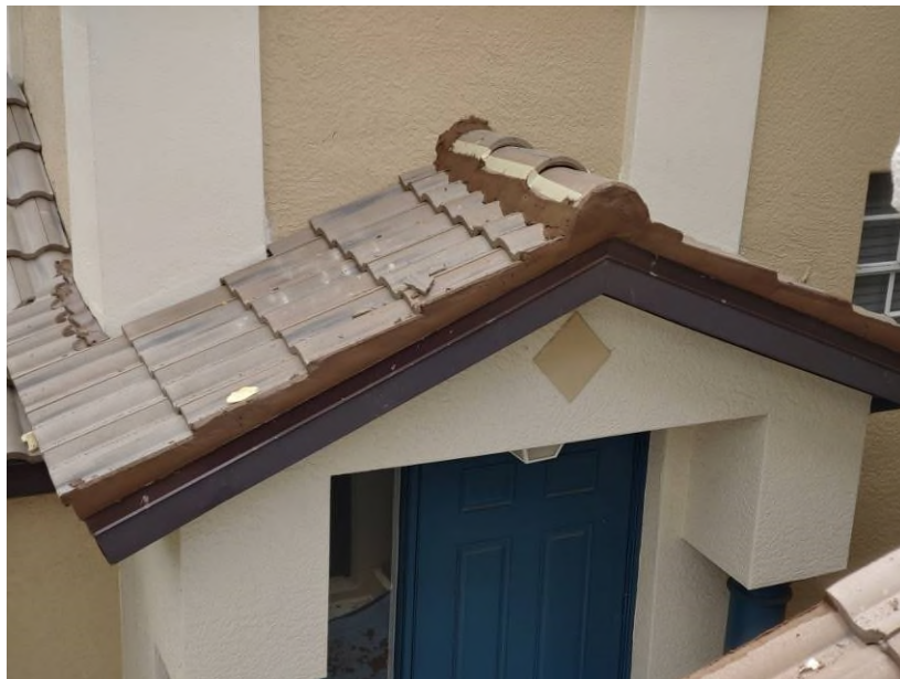
Photograph #2: Mortar adhesive application was in progress surrounding the ridge tiles and hip tiles on building 7840.
