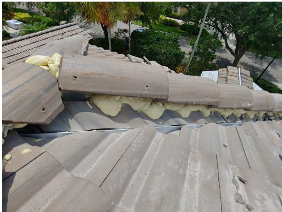
Photograph #6: Roof field, ridge and hip tile installations with polyurethane foam adhesive was in progress on building 21741.
