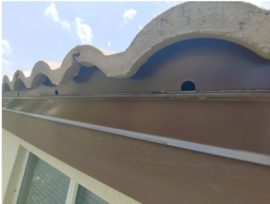
Photograph #7: Bird-stop metal flashing installation was in progress on building 21741.
