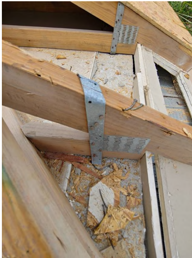
Photograph #15: Existing strap clips on the trusses have the required minimum of 5 nails on building 21821.
