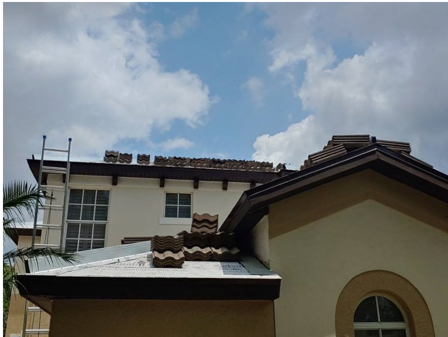
Photograph #11: Roof tiles were set in place for installation on building 21761.
