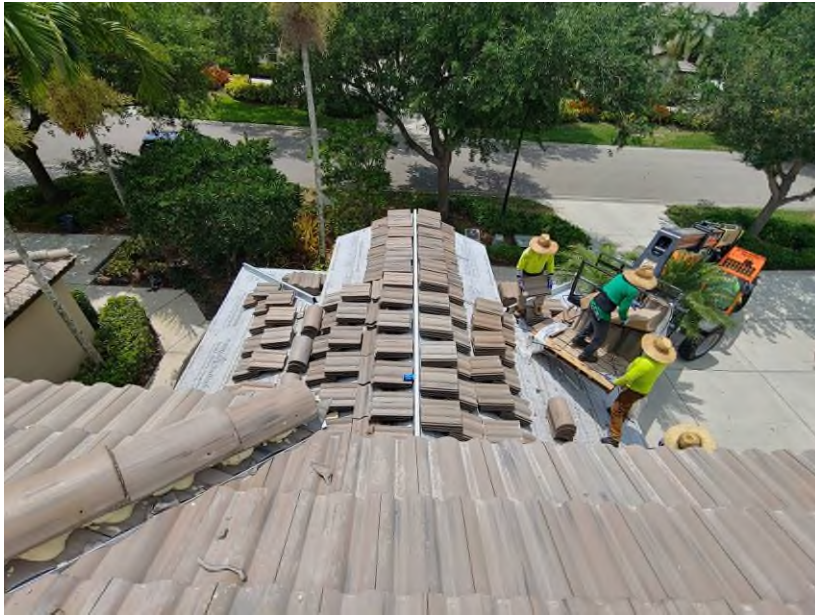
Photograph #9: Roof tiles were set in place for installation on building 21741.
