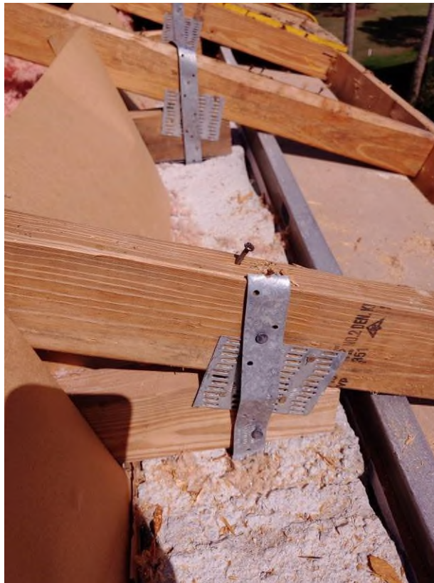
Photograph #7: KEG observed a lack of nails on a few existing straps on building 21721. N8d nails were installed during the site visit to comply with the Florida Building Code.
