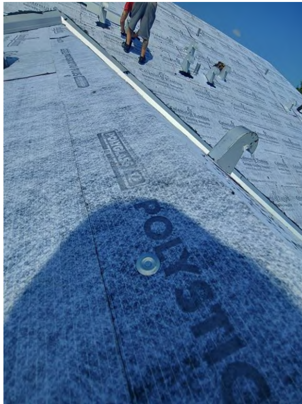
Photograph #5: Contractor must cover all exposed nails with asphalt plastic roofing cement on building 7851.
