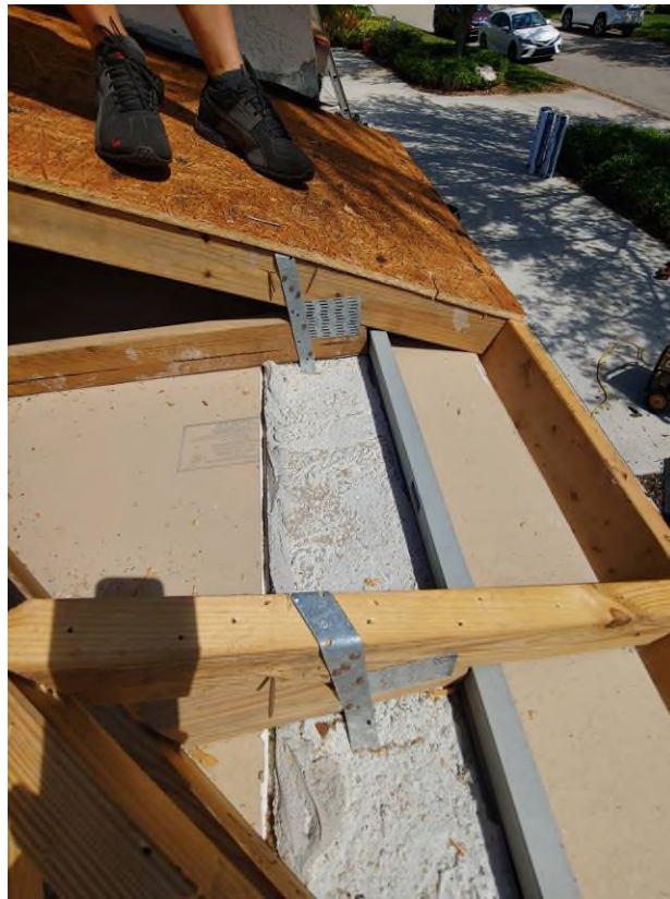
Photograph #7: Existing strap clips on the trusses have the required minimum quantity of nails on building 7861.
