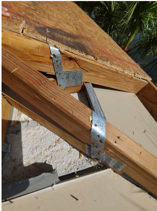
Photograph #2: Existing strap clips on trusses have the required minimum quantity of nails on building 7860.
