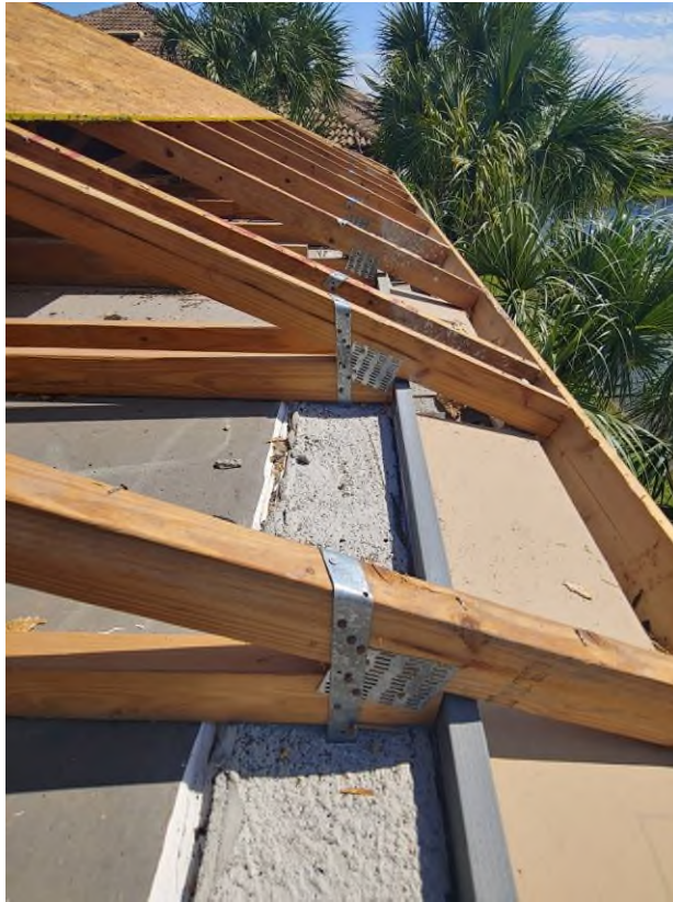
Photograph #11: Existing strap clips on the trusses have the required minimum quantity of nails on building 21740.
