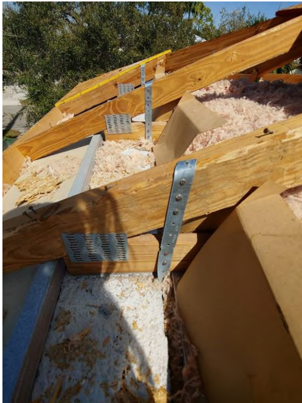
Photograph #12: Existing strap clips on the trusses have the required minimum quantity of nails on building 21740.
