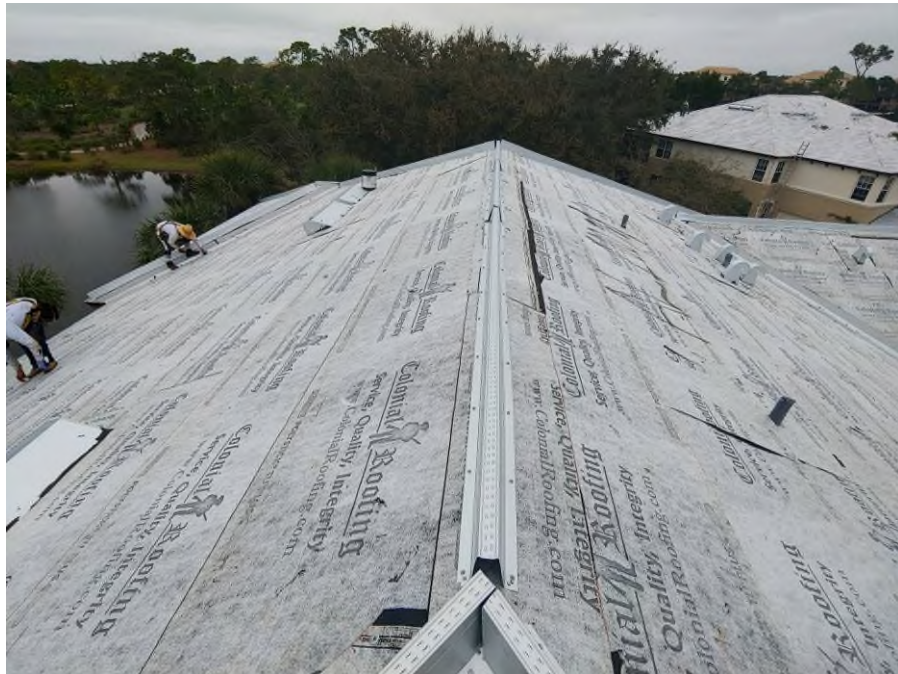
Photograph #6: V-crimp metal valley flashing, and hip/ridge metal channel installations were in progress on building 21700.
