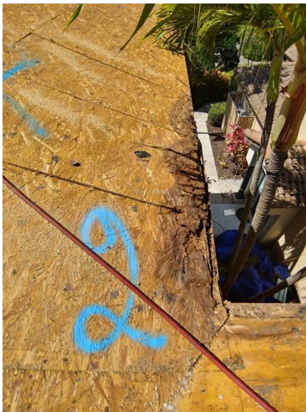
Photograph #26: Rotten fascia and plywood sheathing were observed on building 21761.
