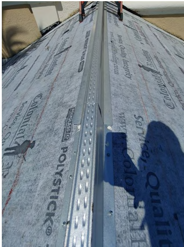
Photograph #9: Hip/ridge metal channel installations were in progress on building 7881.
