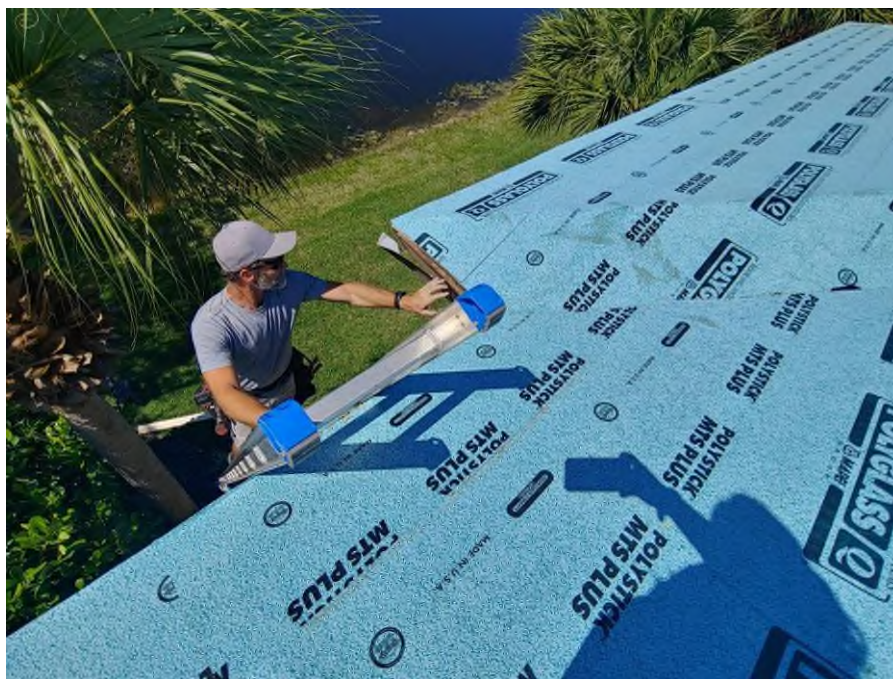
Photograph #21: Fascia repair was observed on building 21770.
