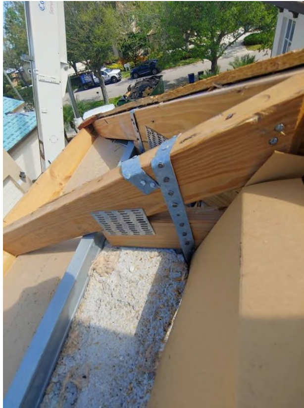
Photograph #15: Existing strap clips on the trusses have the required minimum quantity of nails on building 21770.
