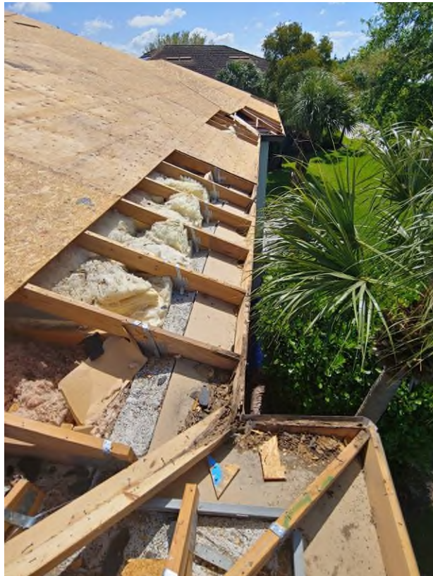
Photograph #16: Rotten fascia and trusses were observed on building 21770.
